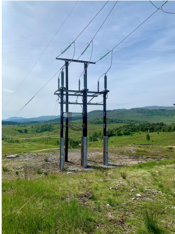
Plate 3.2: Typical Sealing End Structure
