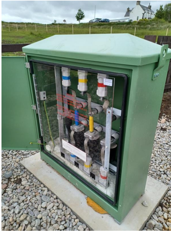
Plate 3.3: Typical Link Pillar
