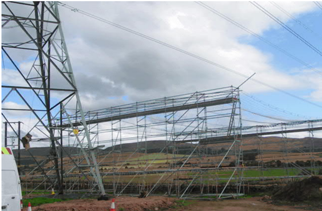
Photo 3.4: Illustrative Image of Temporary Construction Scaffolds
