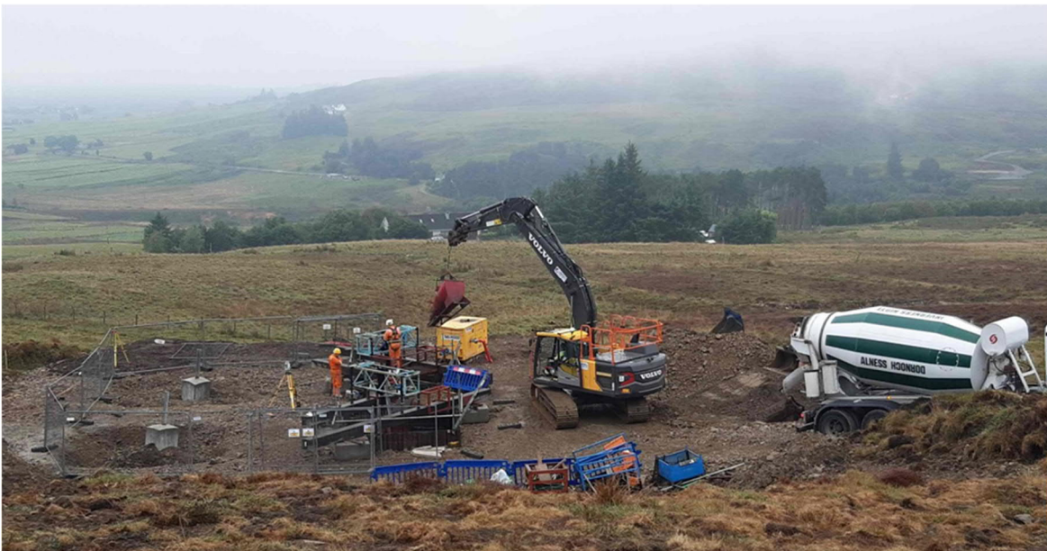
Photo 3.2: Illustrative Image of Tower Foundation Construction
