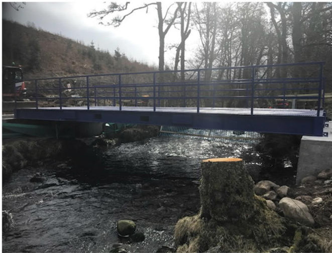
Photograph 10.1 Temporary Clear Span Bridge example
