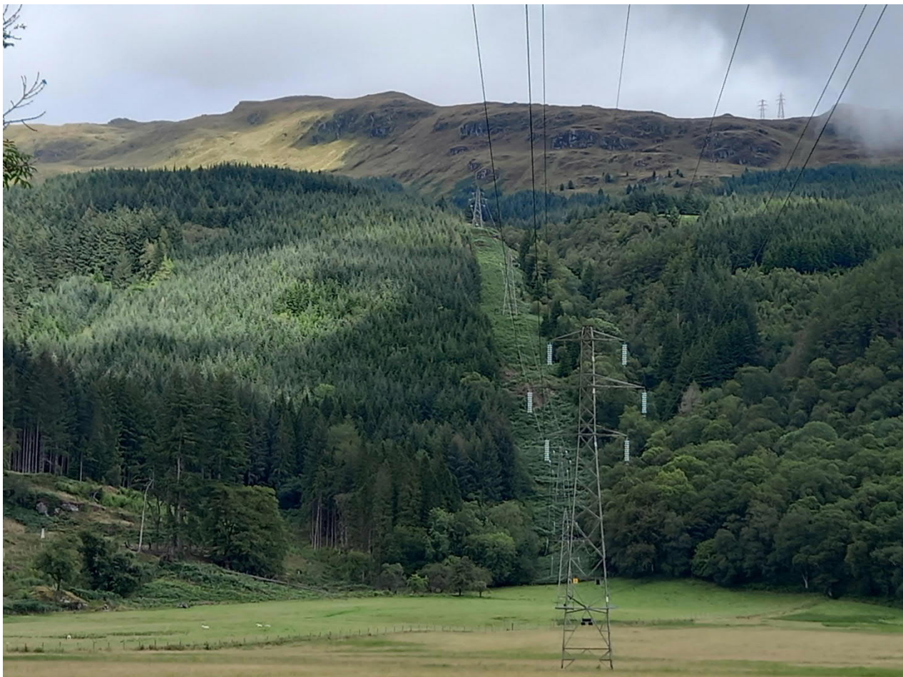
Plate 1 – View looking north up existing wayleave corridor. Proposed new alignment crosses felled area on left. Temporary OHL diversion impacts broadleaved Ancient Woodland (of semi-natural origin) on right.
