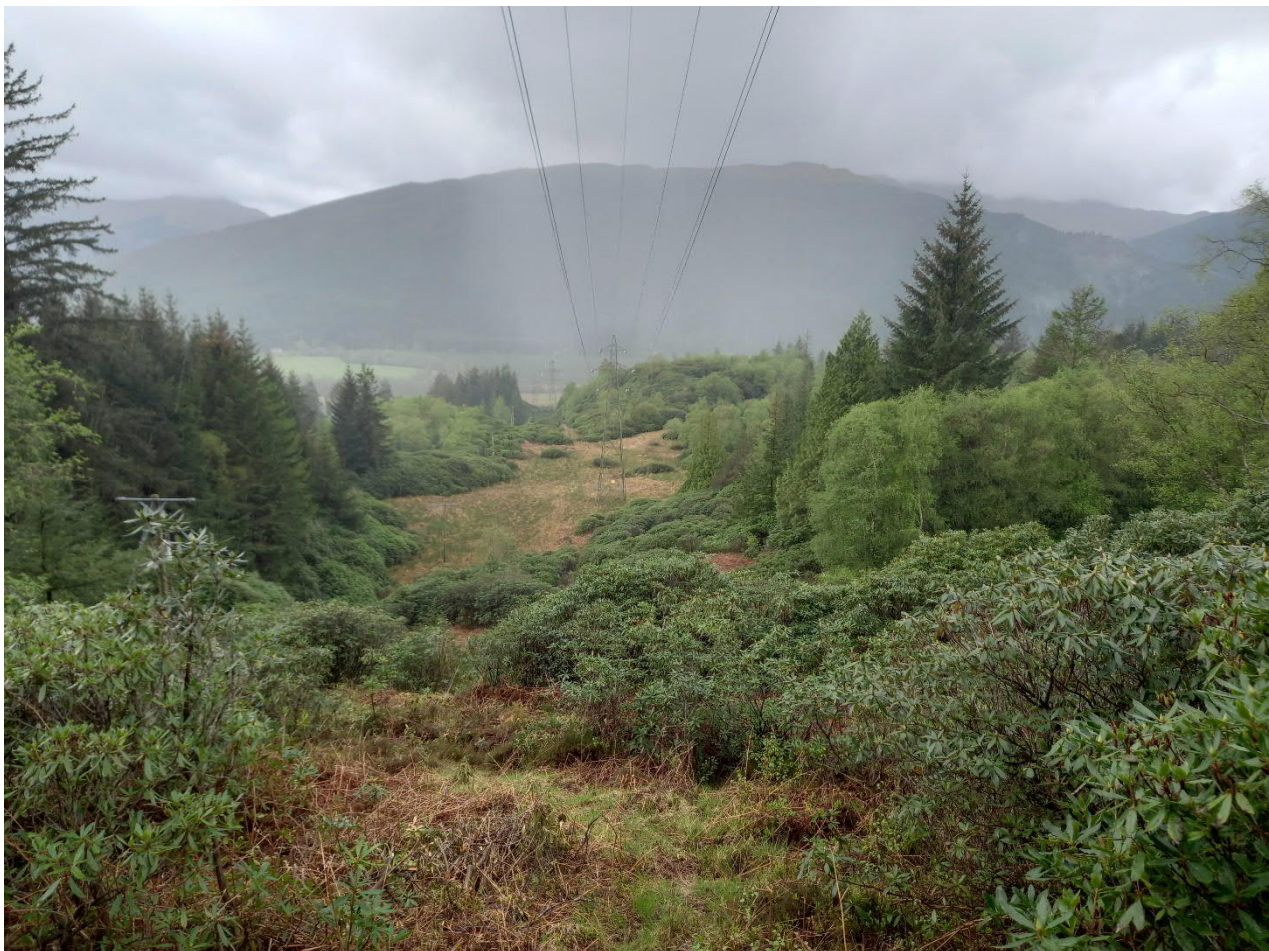
Plate 3 – View from Tower 49 to Tower 50. Birch to be removed from 60m operational corridor. Scattered conifers to be selectively removed within 81m operational corridor.
