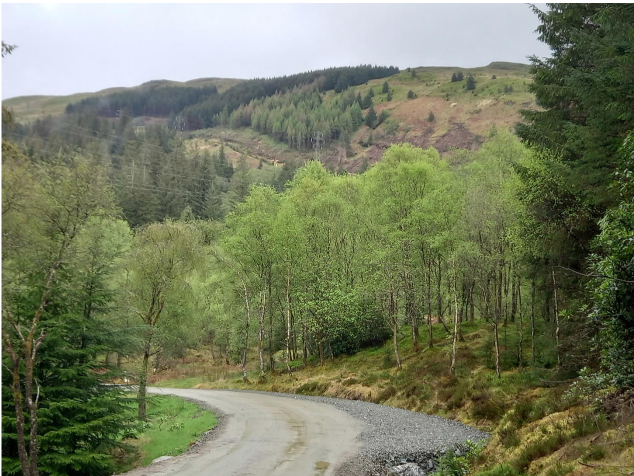
Plate 1 – View from forest road looking NE towards Tower 47. Scheduled sanitation felling can be seen in progress on the hillside.
