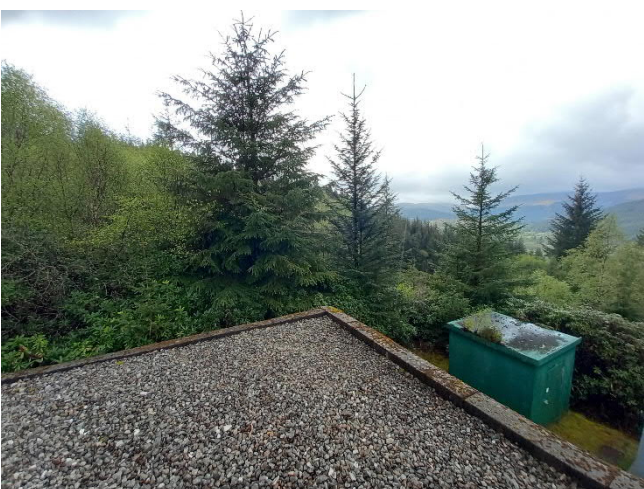
Plate 6 – From Scottish Water covered reservoir looking south. Clearance of birch and conifer regeneration required for track construction.
