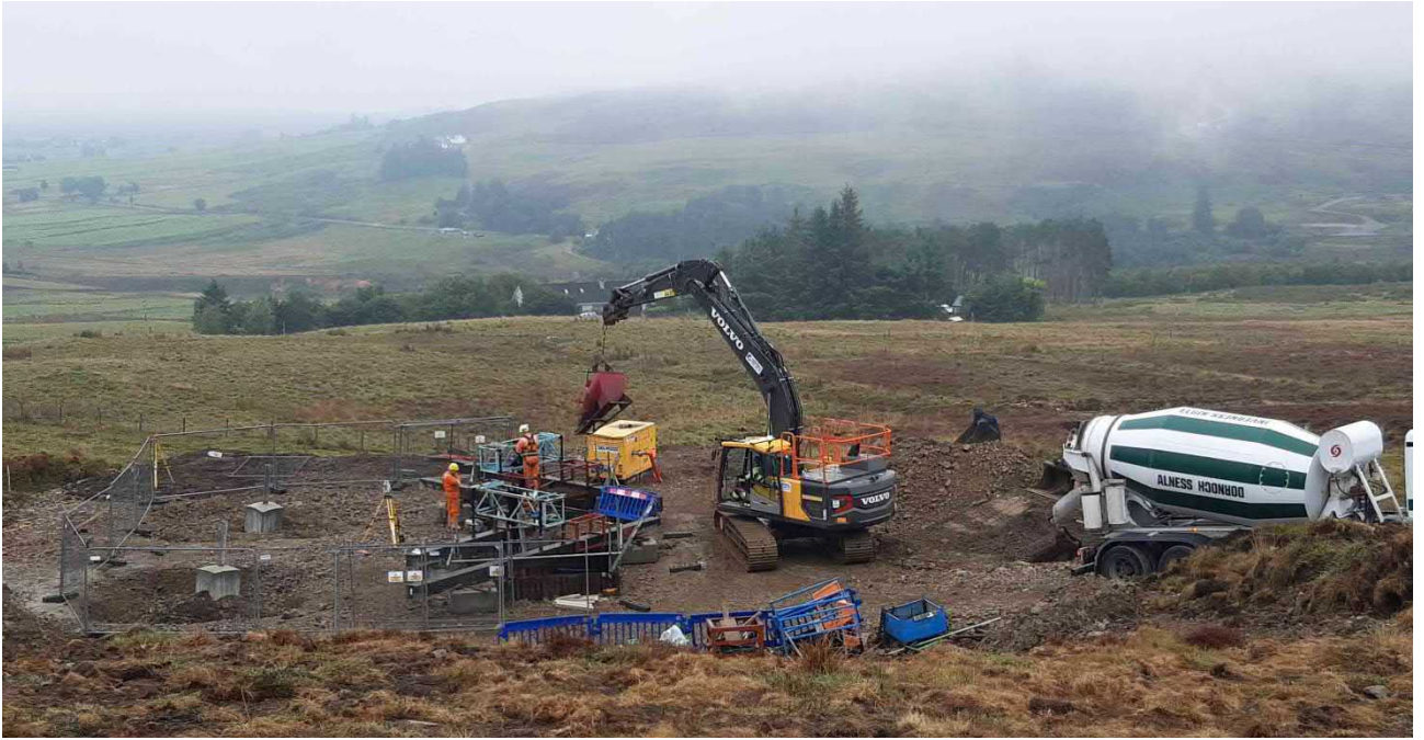
Photo 2.1: Illustrative Image of Tower Foundation Construction
