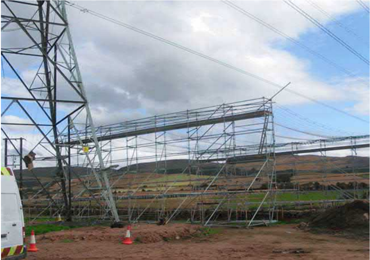
Photo 2.2: Illustrative Image of Temporary Construction Scaffolds
