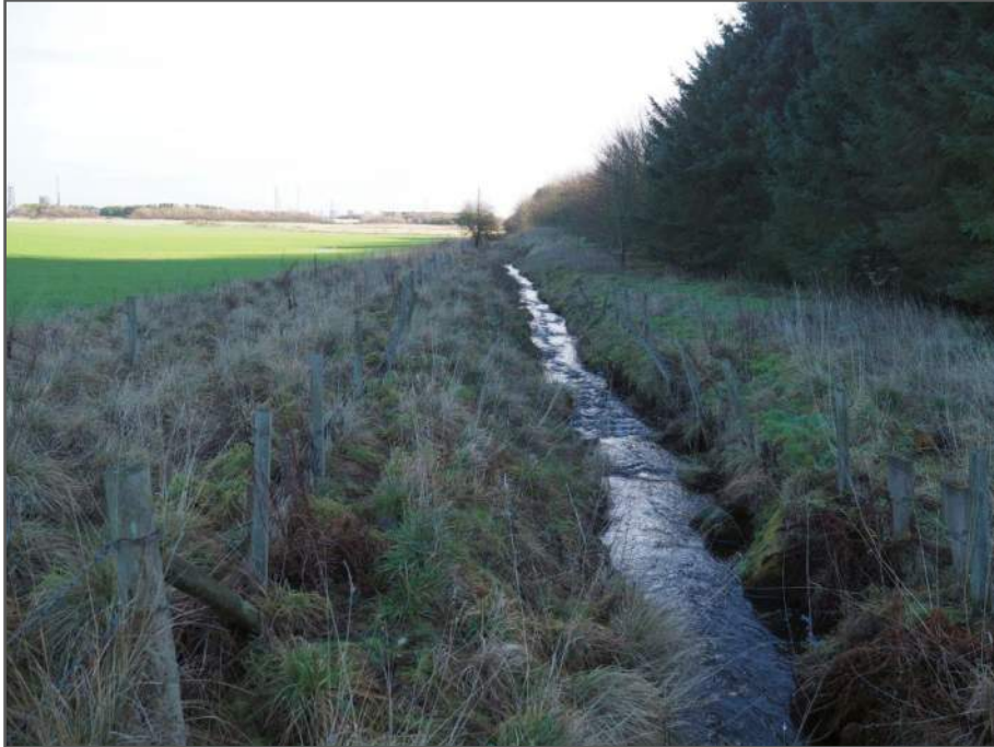
Location 10: Looking downstream along Black Water
