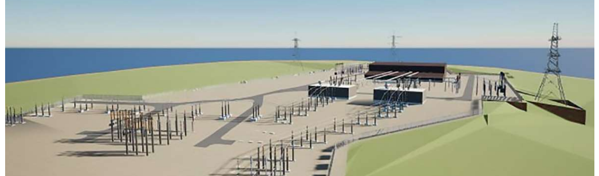
World's First 400kV Green Gas for Grid (G3) Substation - Kintore
