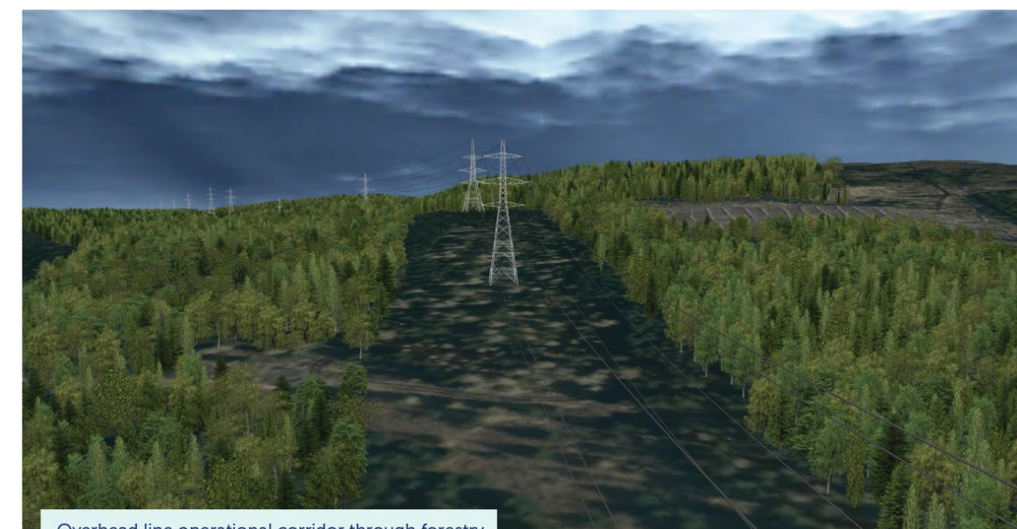
Overhead line operational corridor through forestry
