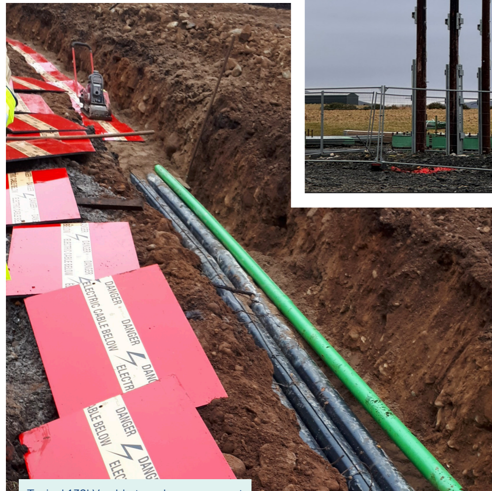
Typical 132kV cable trench arrangement
