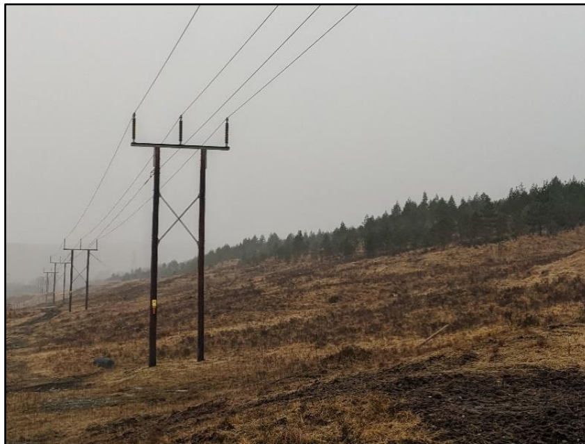
Plate 3.1: Example Trident H-wood poles
