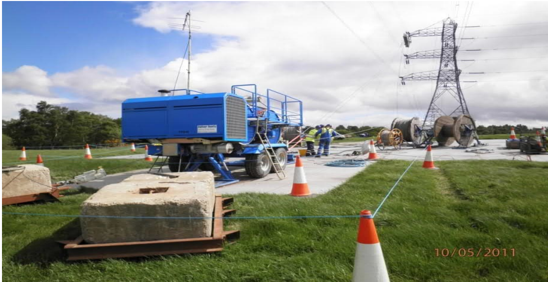
Photograph 3-2 Typical EPZ with equipment set up for reconductoring
