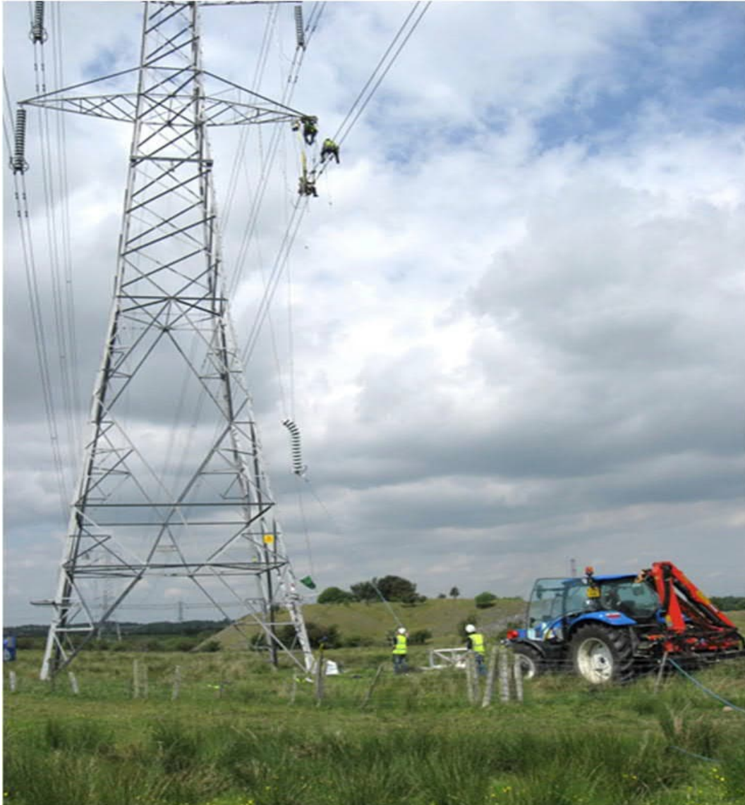
Photograph 3-3 Replacing insulators on an existing OHL tower
