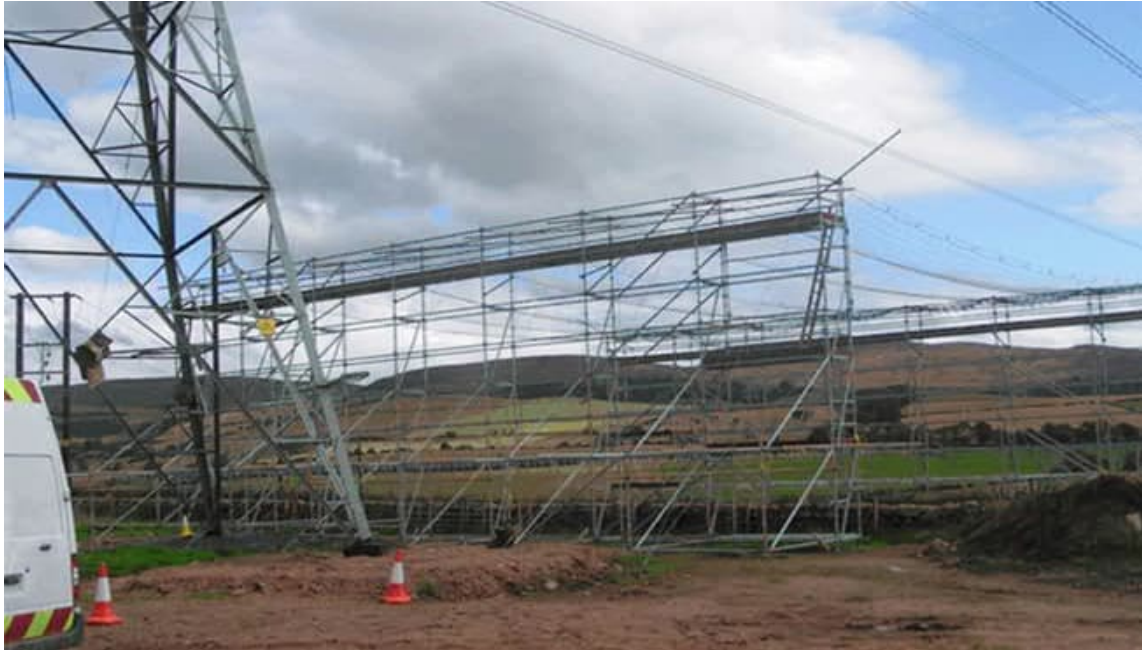
Photograph 3-4 Illustrative image of temporary construction scaffolds
