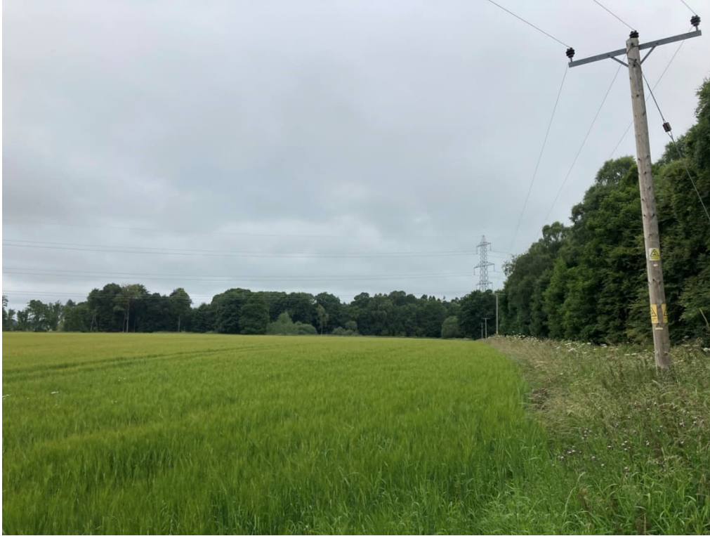
Photograph 4: View along section of 'Trackway Panels' required to access Tower 644 visible beyond the woodland. The track will follow the field edge based on the current design. The field in the central area forms part of the Cardean Roman Camp scheduled area (SM4337).
