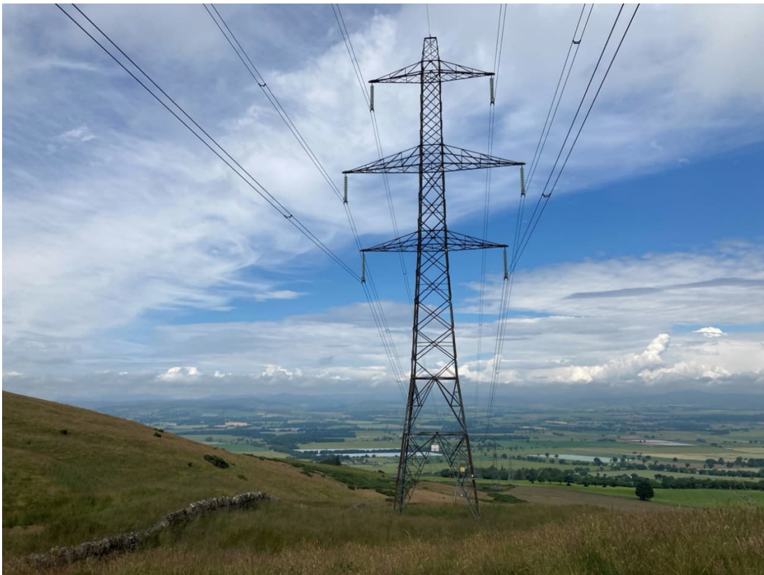
Photograph 13: View north from area of Tower 660 along area of proposed 'New Stone Road' which runs alongside the drystone wall based on the current design.
