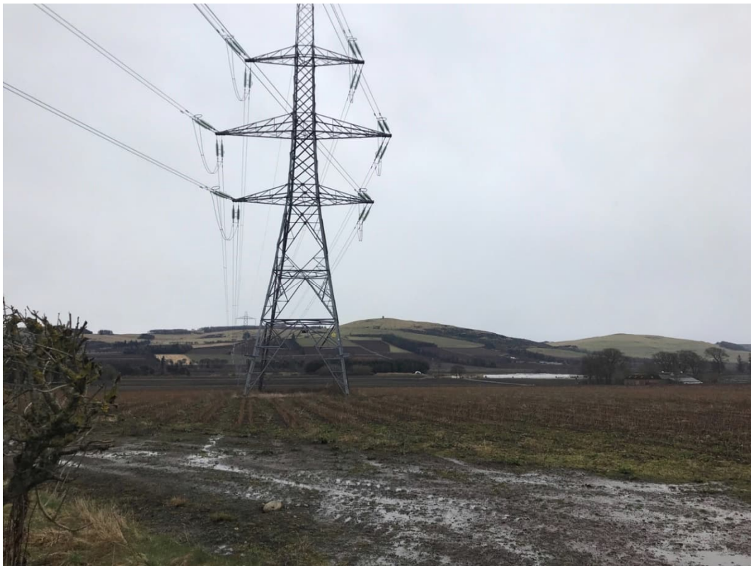
Photograph 8: View south to Tower 648 from proposed bellmouth upgrade. The area is located in close proximity to a possible prehistoric settlement recorded as a cropmark (MPK20338). Access in this area is stated to be 'Trackway Panels' on the current design.
