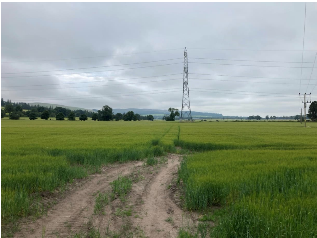
Photograph 10: View southwest towards Tower 653 from area of bellmouth upgrade, and along the alignment of the proposed access which will be by 'Trackway Panels' based on the current design. The former farmstead of Myreside (AECOM001) was located in the area of Tower 653.
