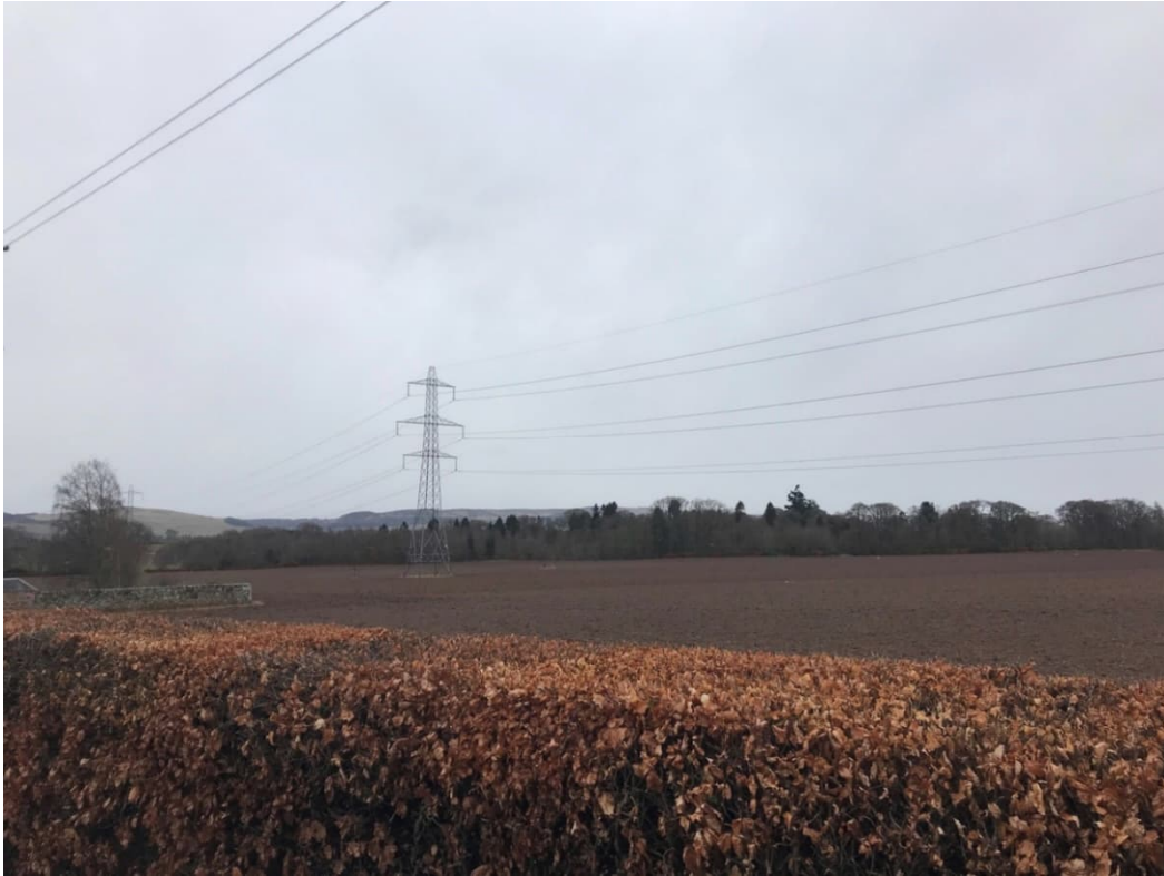
Photograph 1: View of the scheduled Cardean Roman Camp (SM4337) from the east showing the operational OHL and the tower that sits within the west border of the scheduled area. The nearby scheduled Cardean Roman Fort (SM2306) occupies the agricultural land in front of the trees in the right half of the image.
