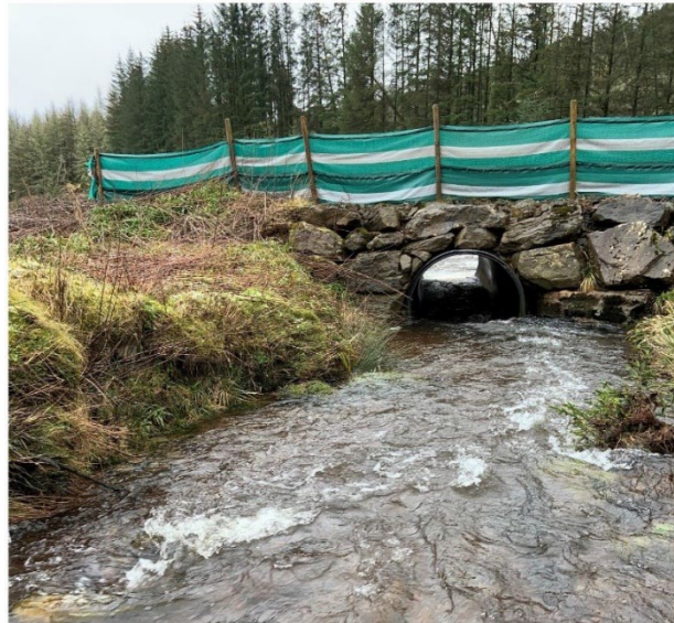
Plate 3.5: Silt Fencing at Watercourse Crossing
