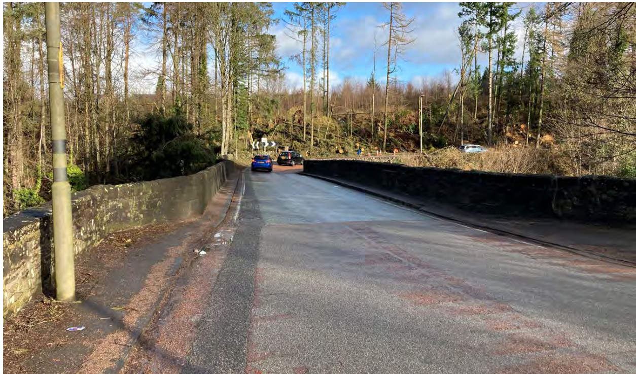
3d. Cross River Teith Bridge – Bridge will need to be cleared by BEAR Scotland.
