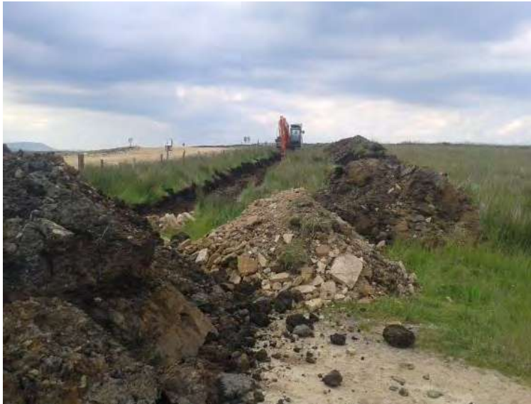
Plate 3.2: Stockpile and drainage ditch (under construction)
