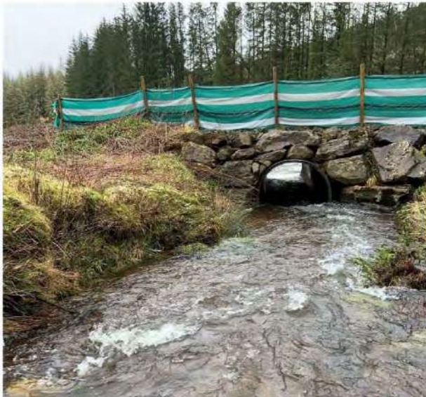
Plate 3.5: Silt Fencing at Watercourse Crossing
