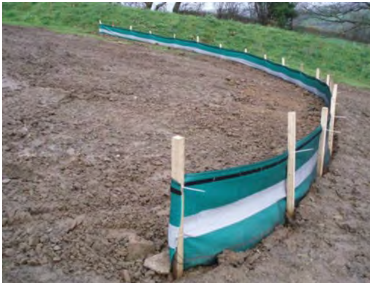
Plate 3.5: Silt Fencing at Watercourse Crossing
