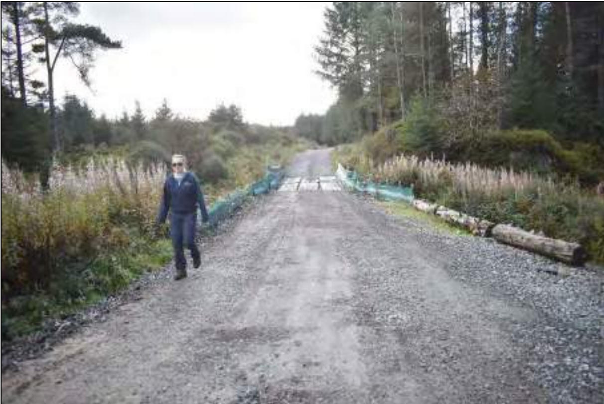
Plate 15: Location of bridge CR03, facing southwest
