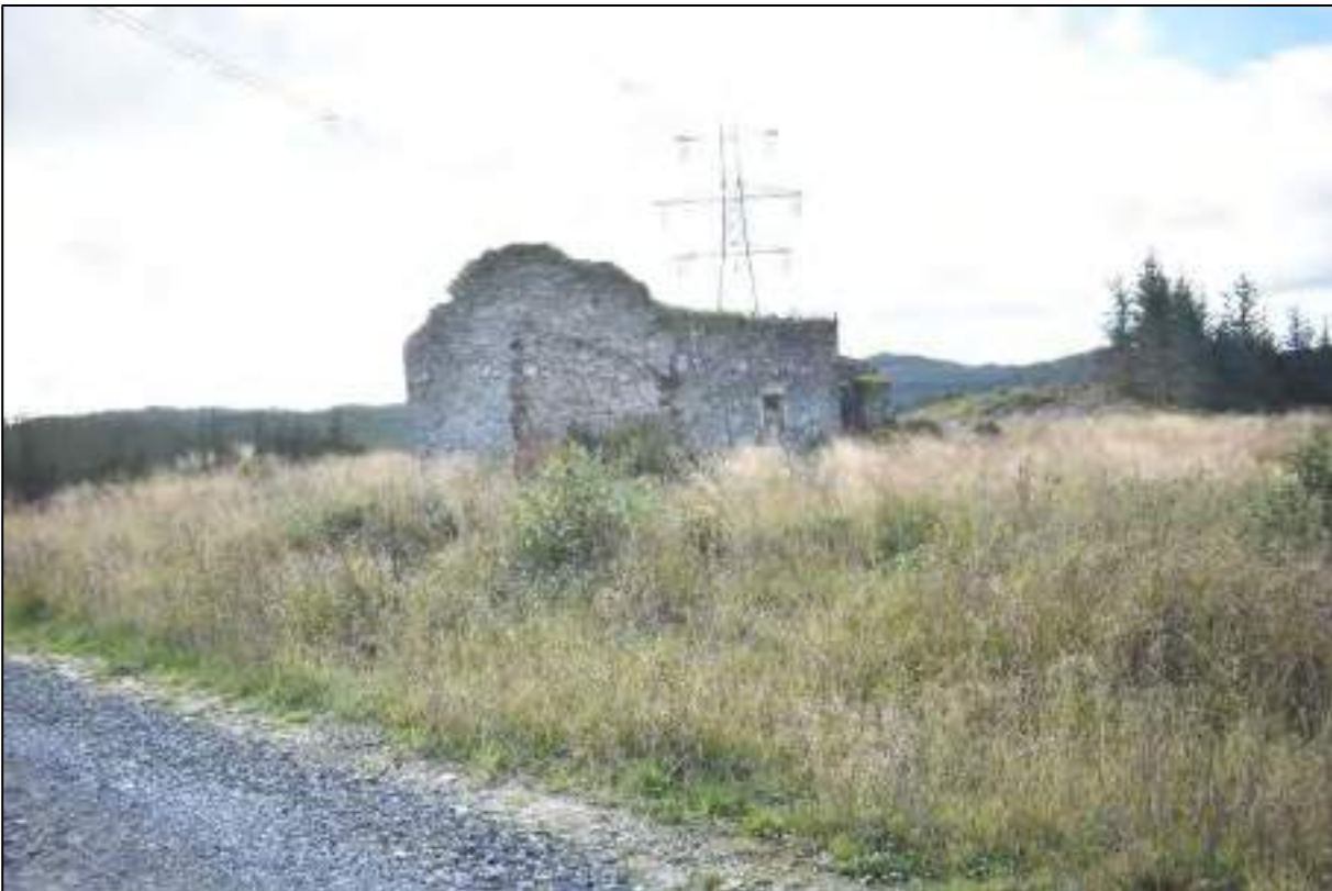
Plate 14: Location of settlement asset CR04, facing southwest
