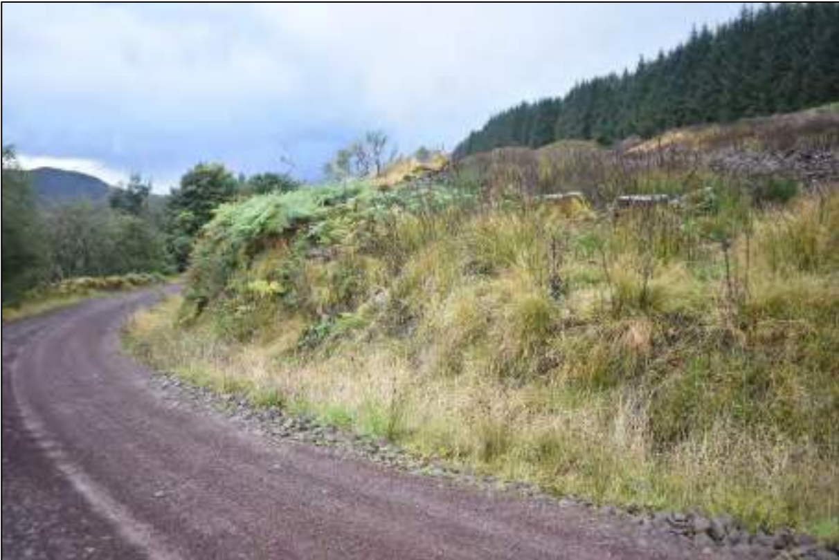
Plate 5: Overgrown drystone dyke AS03, facing southwest
