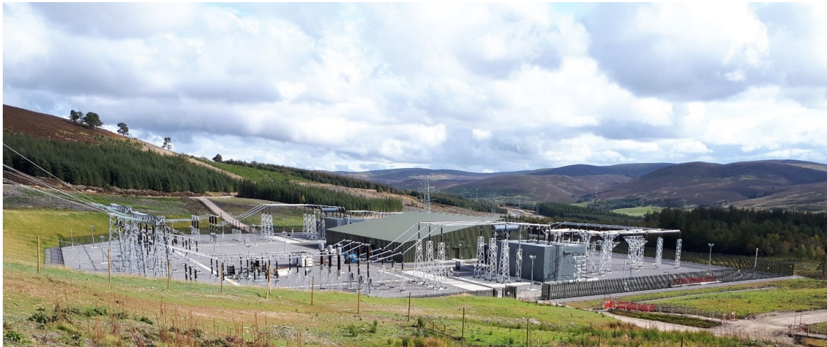
Photo 1.1: Typical Substation design
