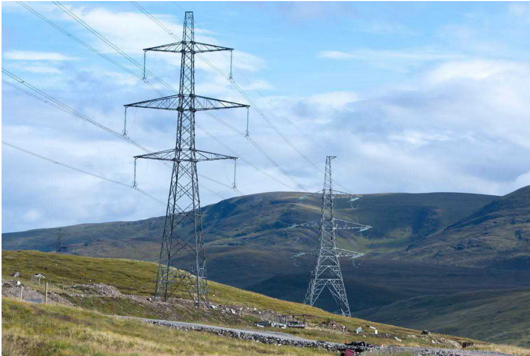
Plate 2.1 – Typical SSE400 steel lattice tower design
