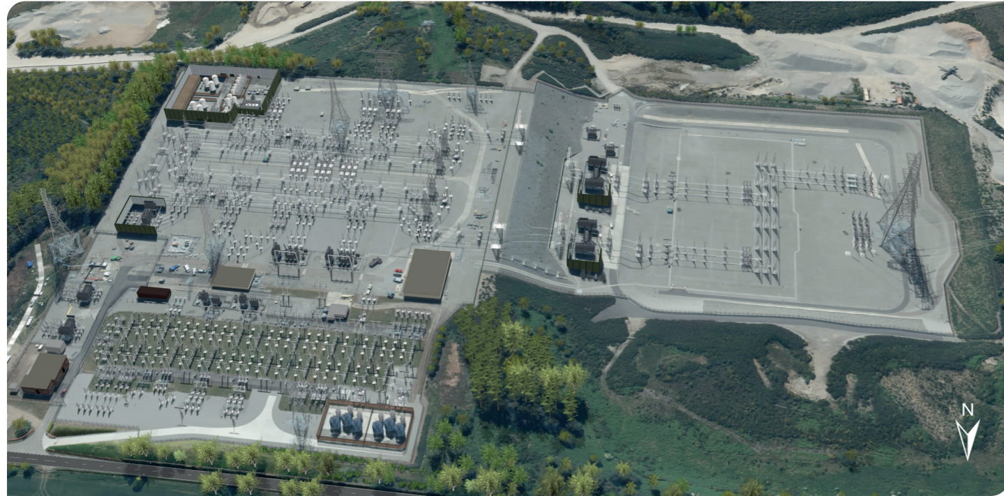
Beaulieu Substation - Before
