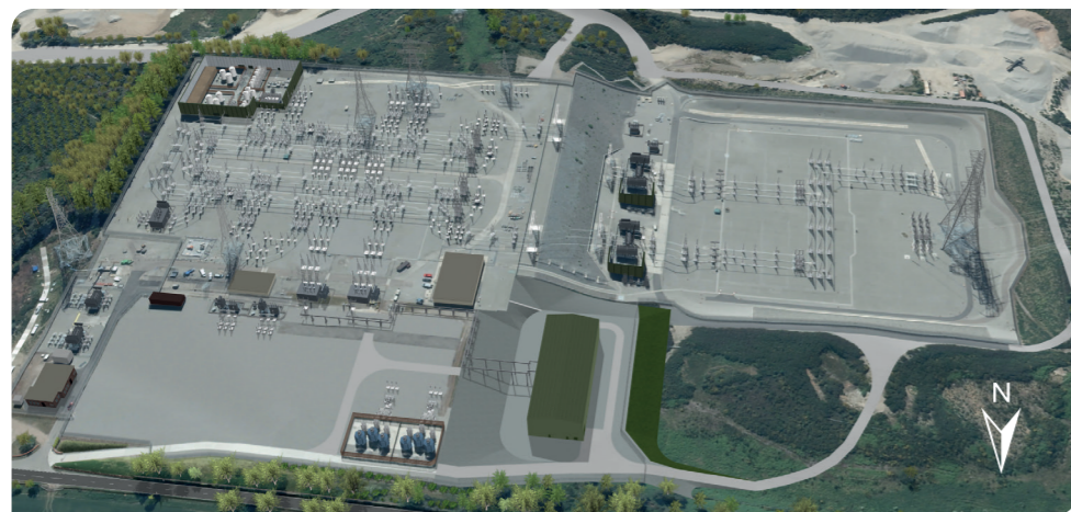
Beauly Substation - After
