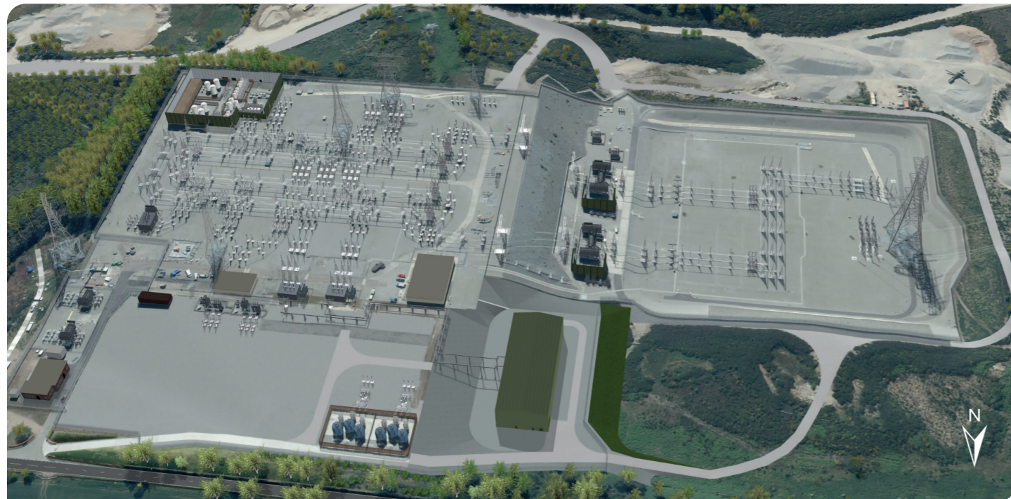
Beaulieu Substation - After
