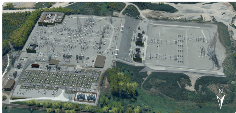
Beauly Substation - Before
