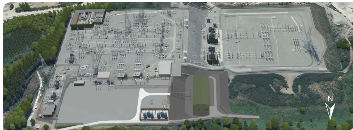
Beauly Substation - After
