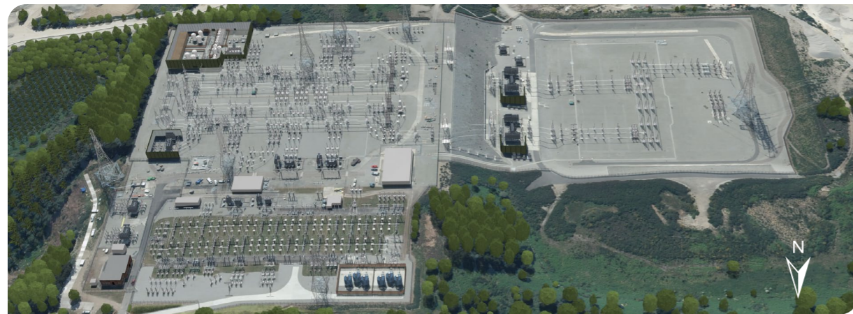
Beauly Substation - Before
