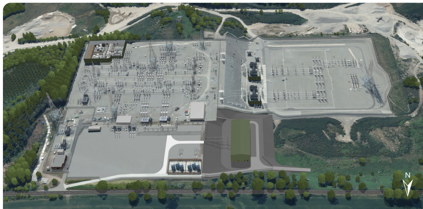
Beaulieu Substation - After
