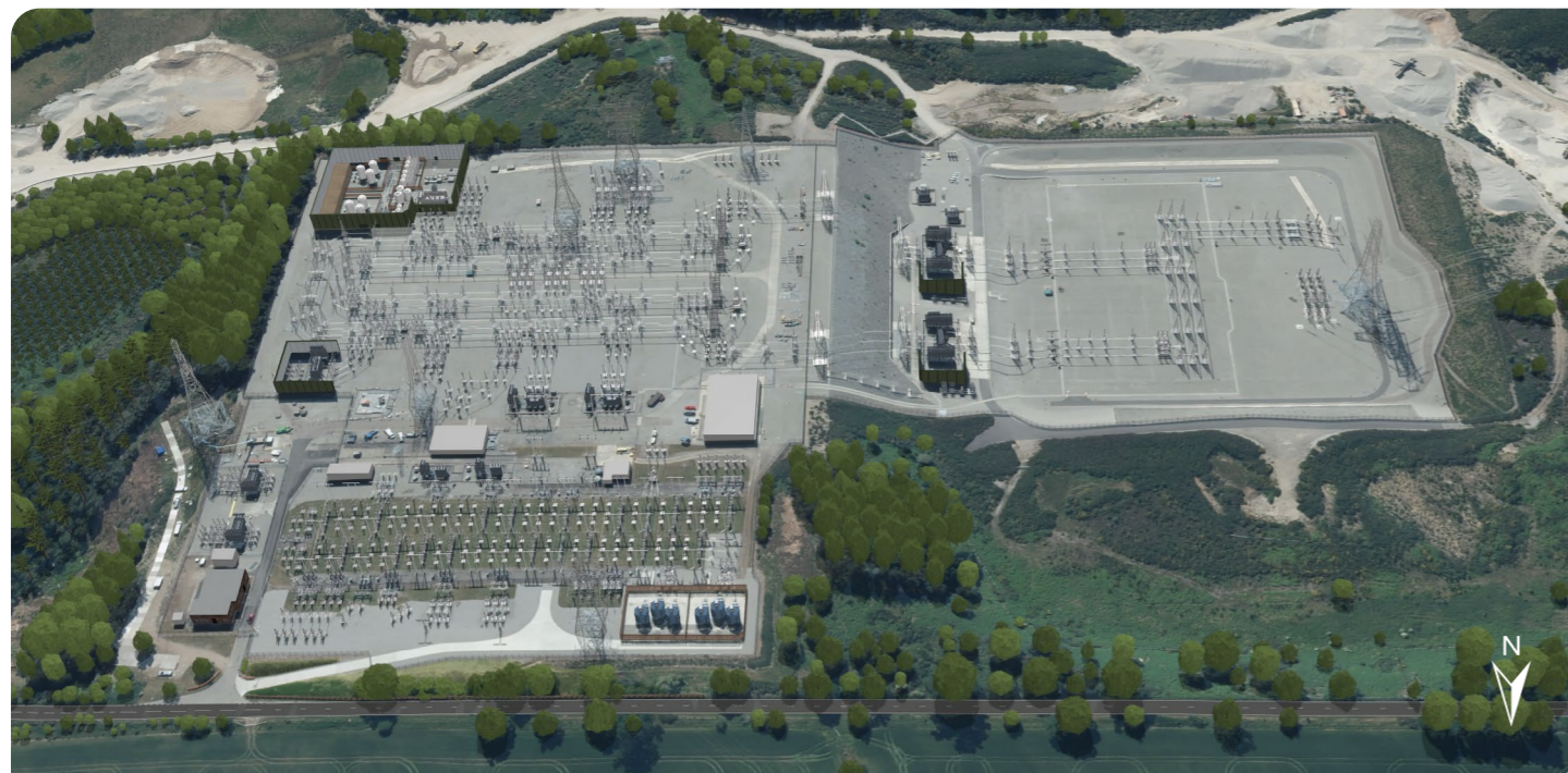
Beaulieu Substation - Before
