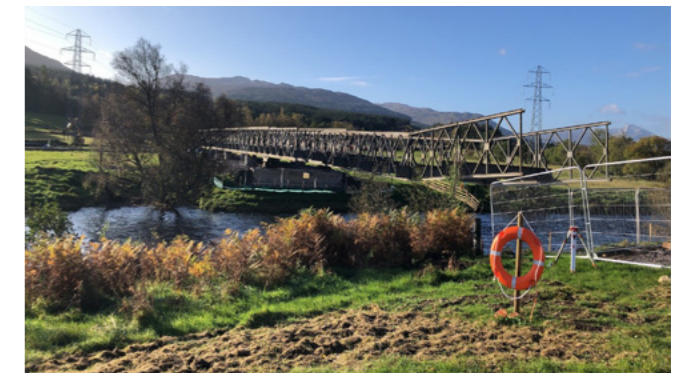
Example of a Bailey bridge used on a nearby SSEN Transmission project at Killin which would be used for the haul road crossing the Keir Burn.
