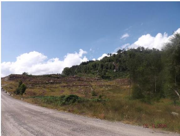
Photo 5: Recently felled woodland along wind farm access
