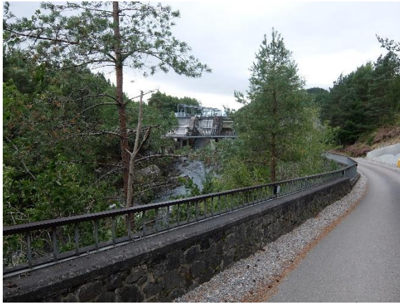
Photo 1: View westward of Dundreggan Dam
