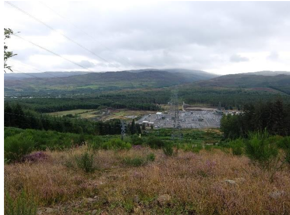
Photo 4: View southward over Fort Augustus substation
