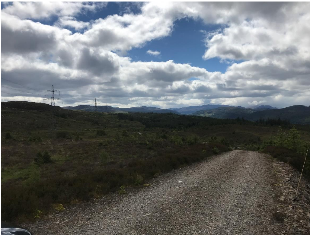
Photograph 6: General view of the existing access track to be upgraded at the western end of the Site near the substation.
