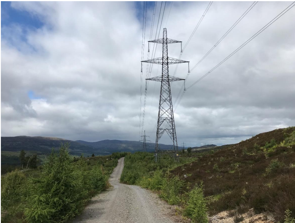
Photograph 8: General view of the substation area (right of image) facing west.
