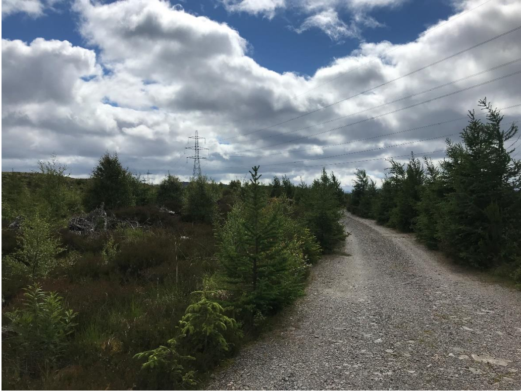
Photograph 7: General view of the substation area (left of image) and existing access track in the area, facing west.
