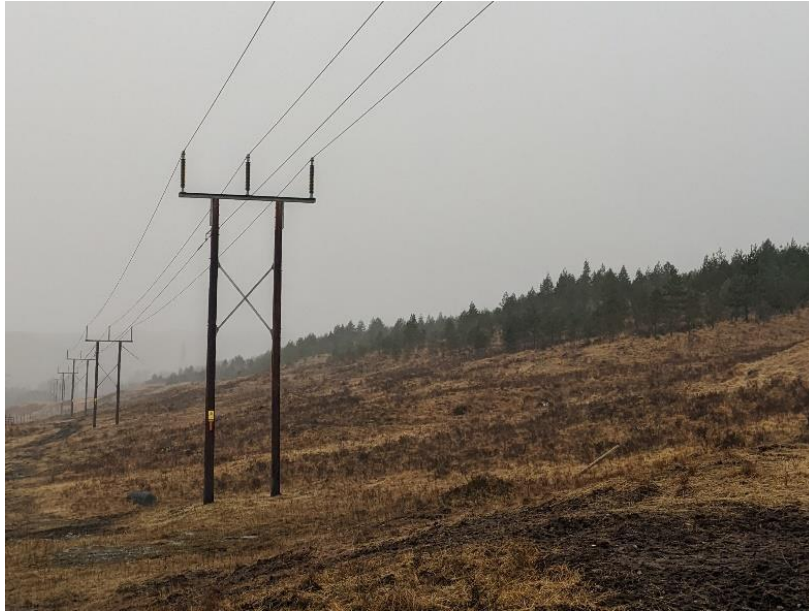
Plate 2.1 – Typical wooden trident pole design
