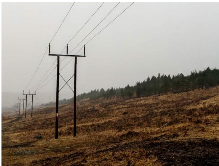
Plate 2.1 – Typical wooden trident pole design
