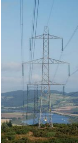
Plate 3.4: Example Steel Lattice Tower
