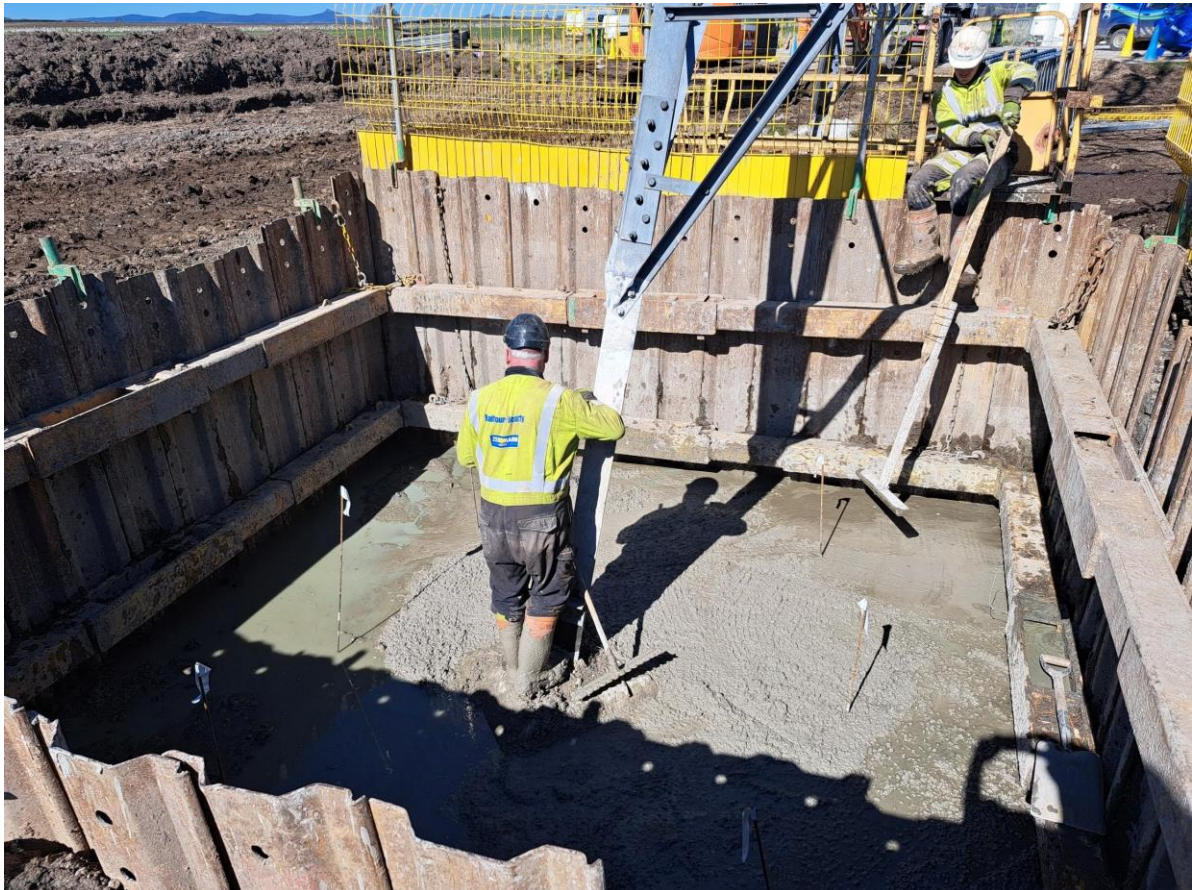
Plate 3.3: Illustrative Image of Tower Foundation Construction
