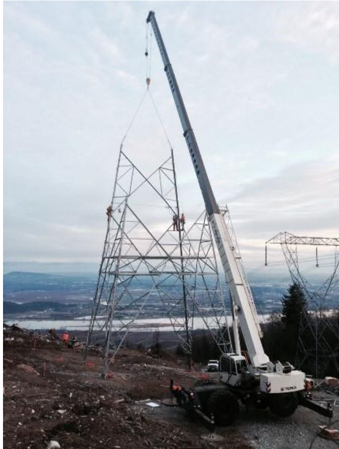
Conductor Stringing – Steel Lattice Towers
