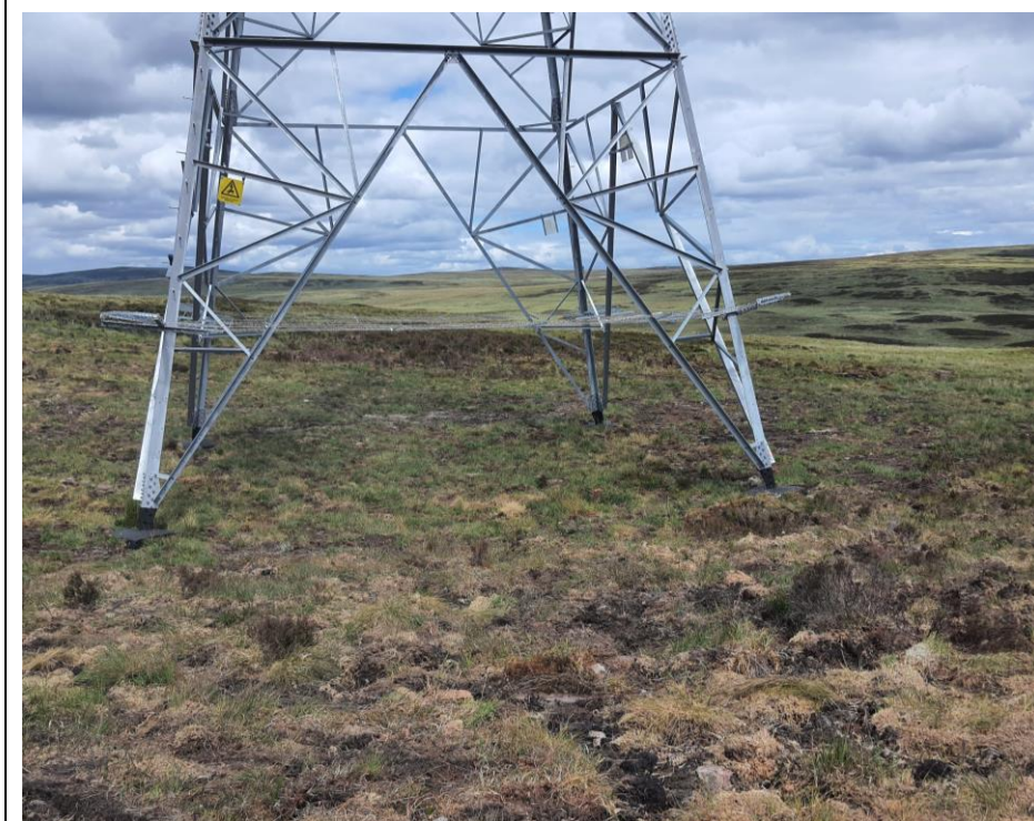
Photo 2: Example of reinstatement around tower foundations.
