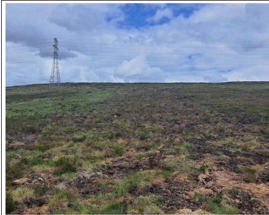
Photo 1: Reinstatement of temporary track using turves.
