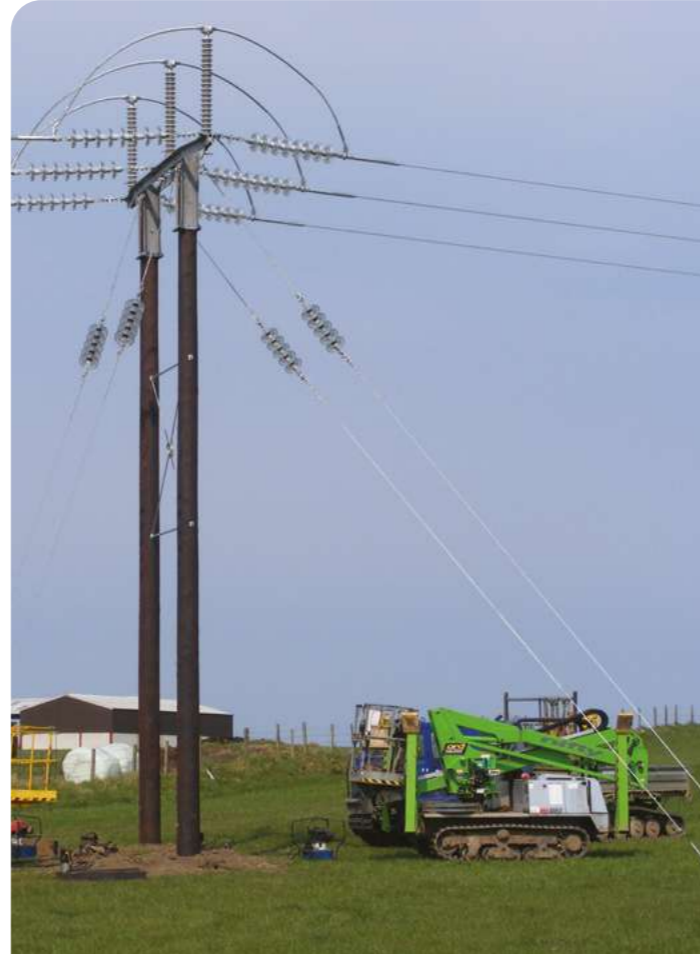
Above is a typical example of an angle wood pole which requires additional stays. Note that stays are not usually required on non-angle poles unless ground or weather conditions dictate.
