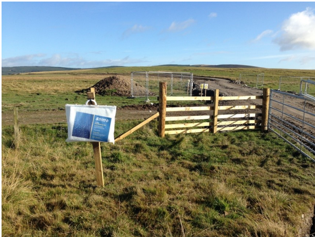
Plate 3.8: Spill Kit Provision on Site
