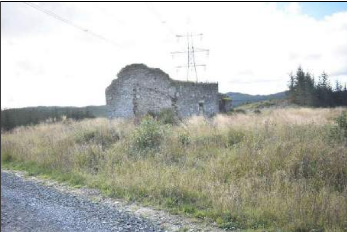
Plate 14: Location of settlement asset CR04, facing southwest
