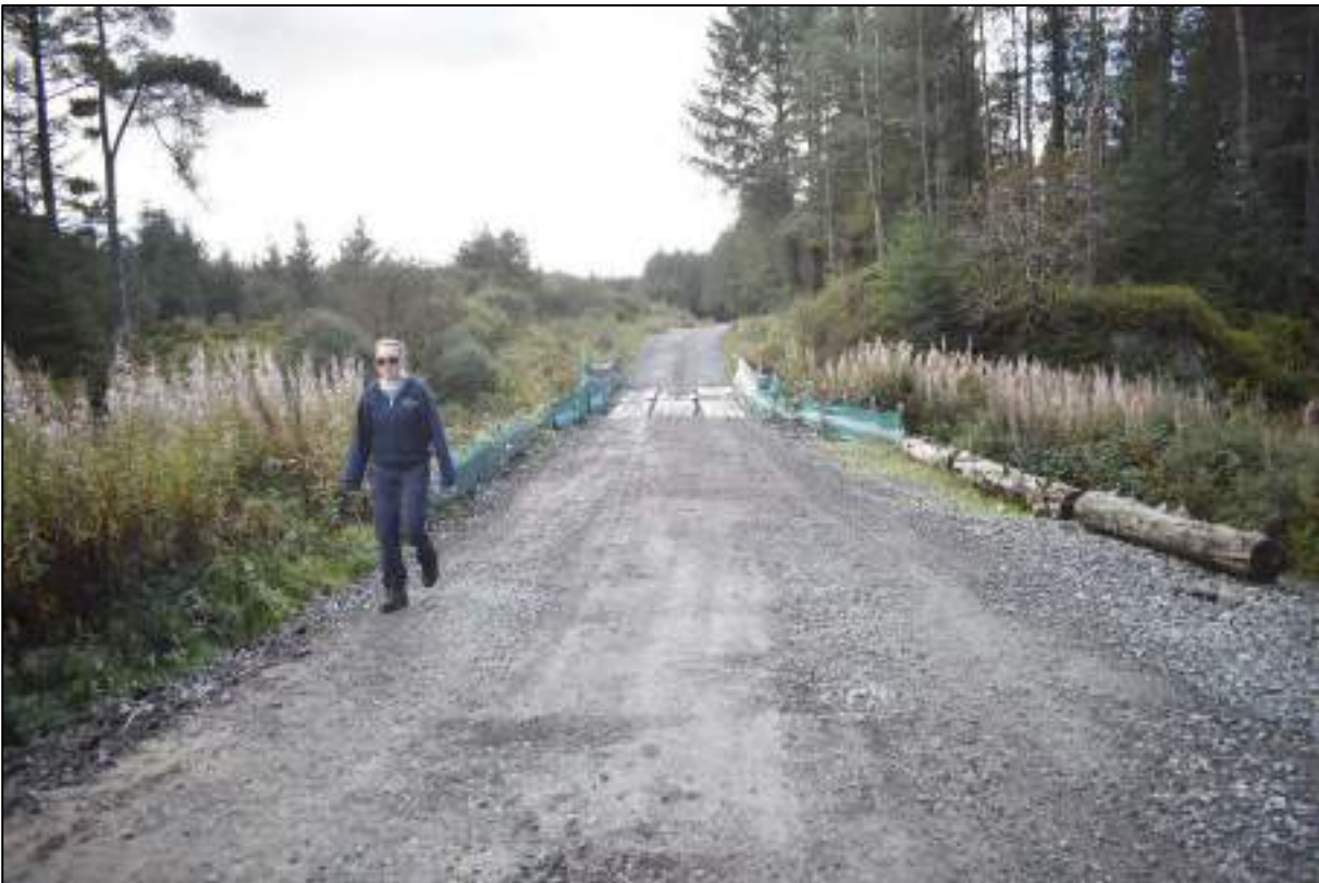
Plate 15: Location of bridge CR03, facing southwest
