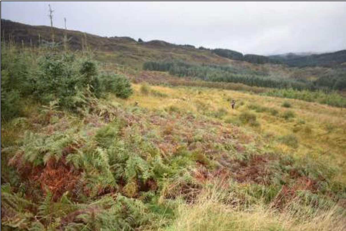
Plate 3: Overgrown drystone dyke AS01, facing northwest
