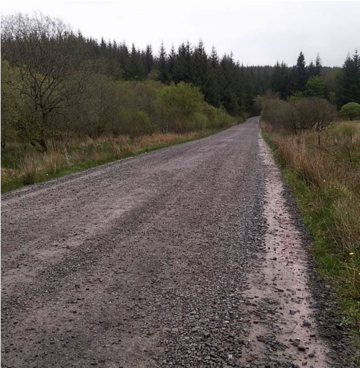
Plate 13 – Shows view of the existing access track from the bellmouth facing east towards the Project. This track has recently been upgraded for the Inveraray to Crossaig OHL project with suitable clearance on either side of the track, self-seeded broadleaves can be seen next to the roadside ditch within 10 m from the track's centreline.
