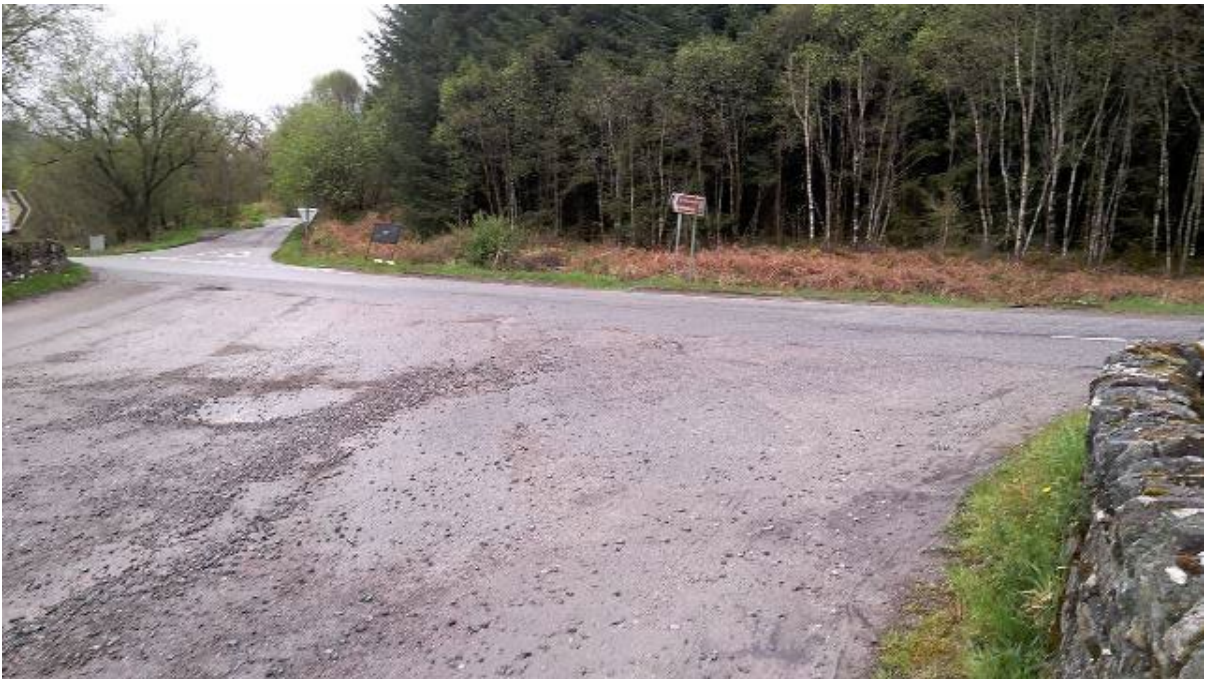
Plate 12 – A view of the bellmouth of the existing access road looking out onto the A816. There is a wide turning circle present.
