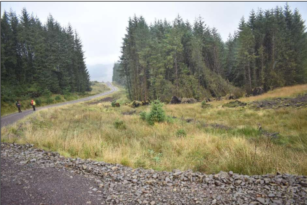
Plate 4: Landscape view of An Suidhe OHL tie-in, facing northeast
