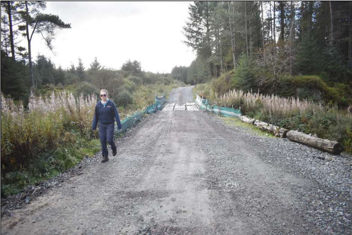
Plate 15: Location of bridge CR03, facing southwest
