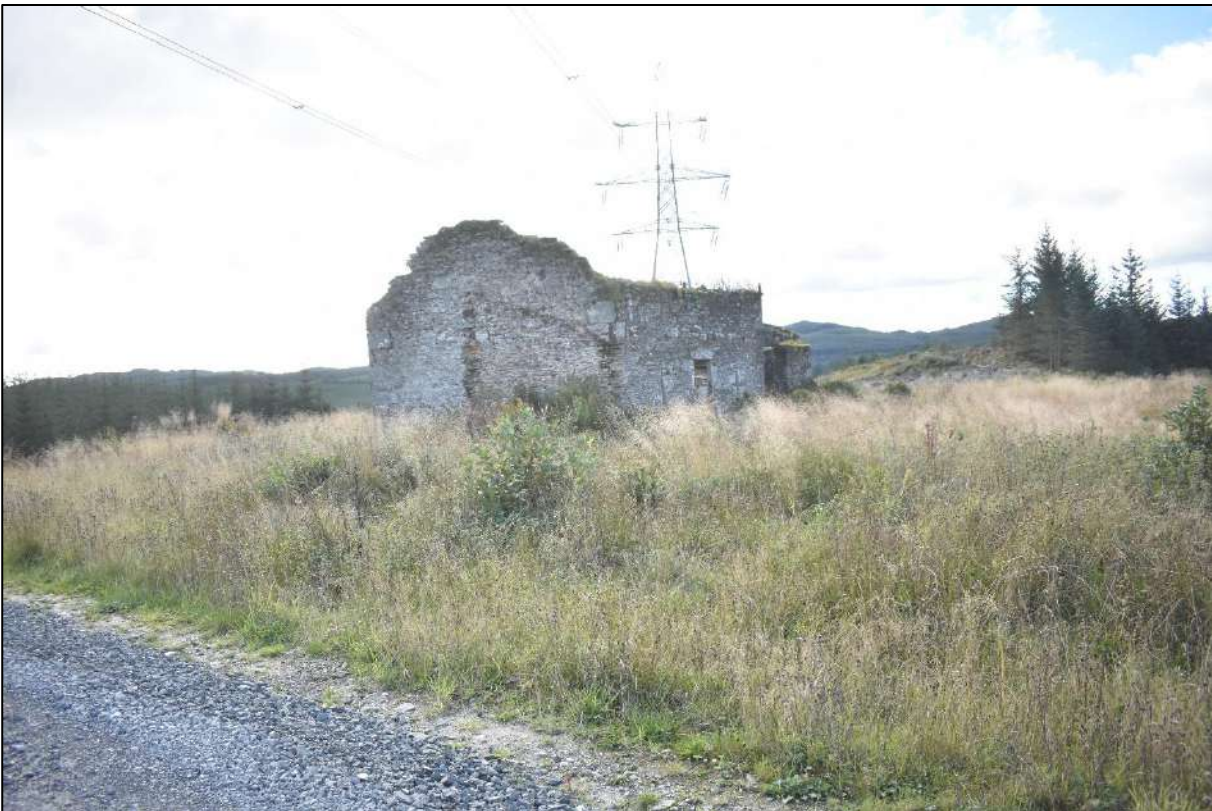
Plate 14: Location of settlement asset CR04, facing southwest
