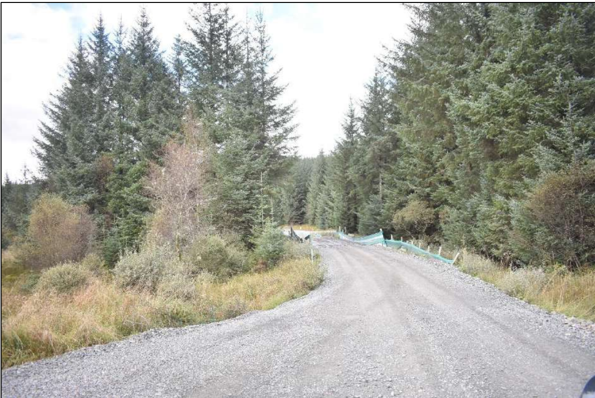
Plate 16: Location of bridge CR05, facing northwest
