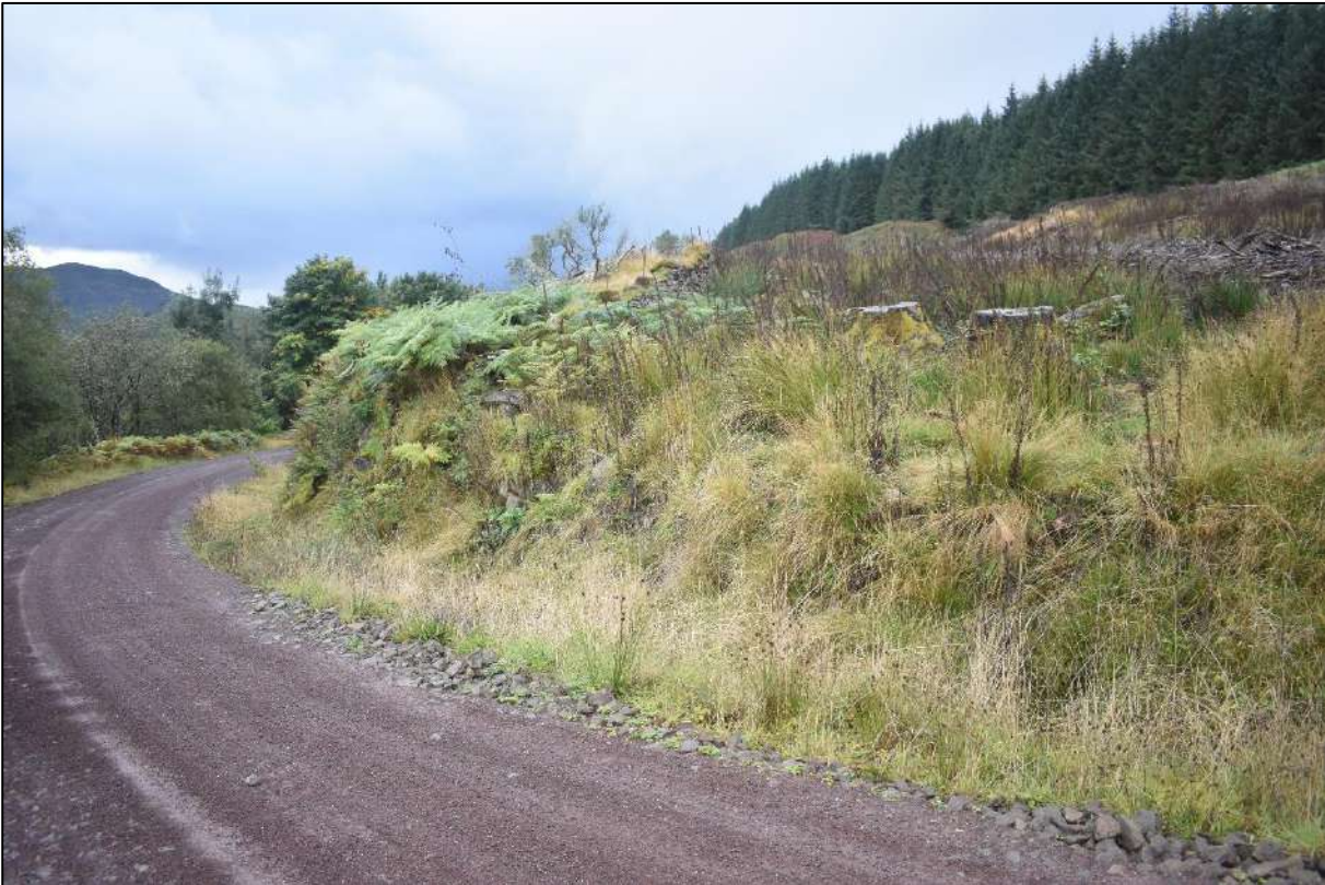
Plate 5: Overgrown drystone dyke AS03, facing southwest
