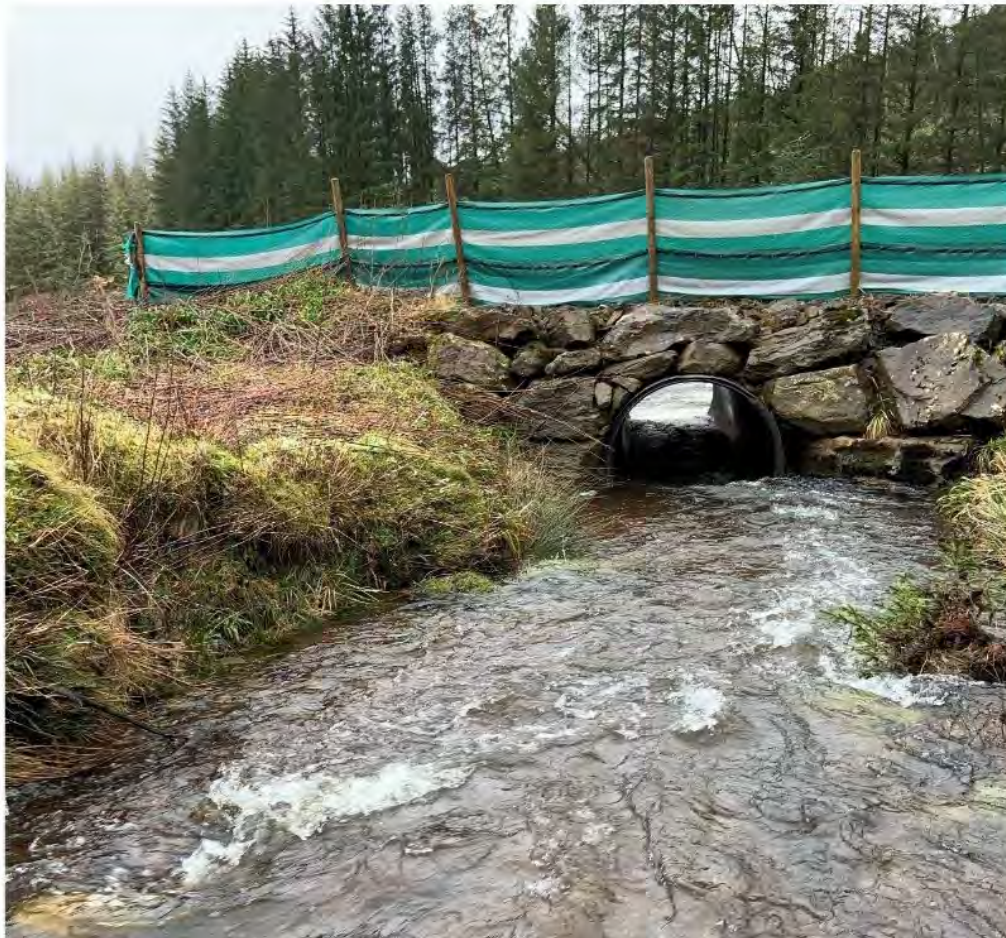
Plate 3.4: Silt Fencing at Watercourse Crossing
