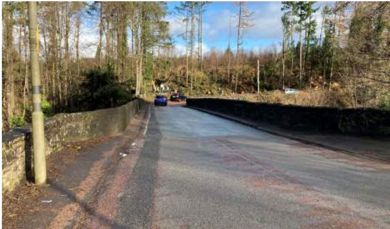
3d. Cross River Teith Bridge – Bridge will need to be cleared by BEAR Scotland.
