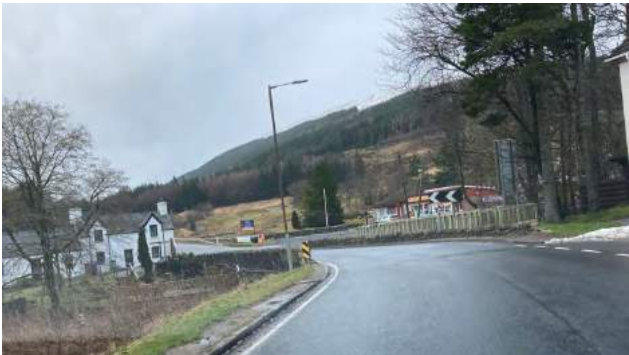
5d. Cross bridge at the Green Welly Stop. Structure to be cleared by BEAR Scotland.
