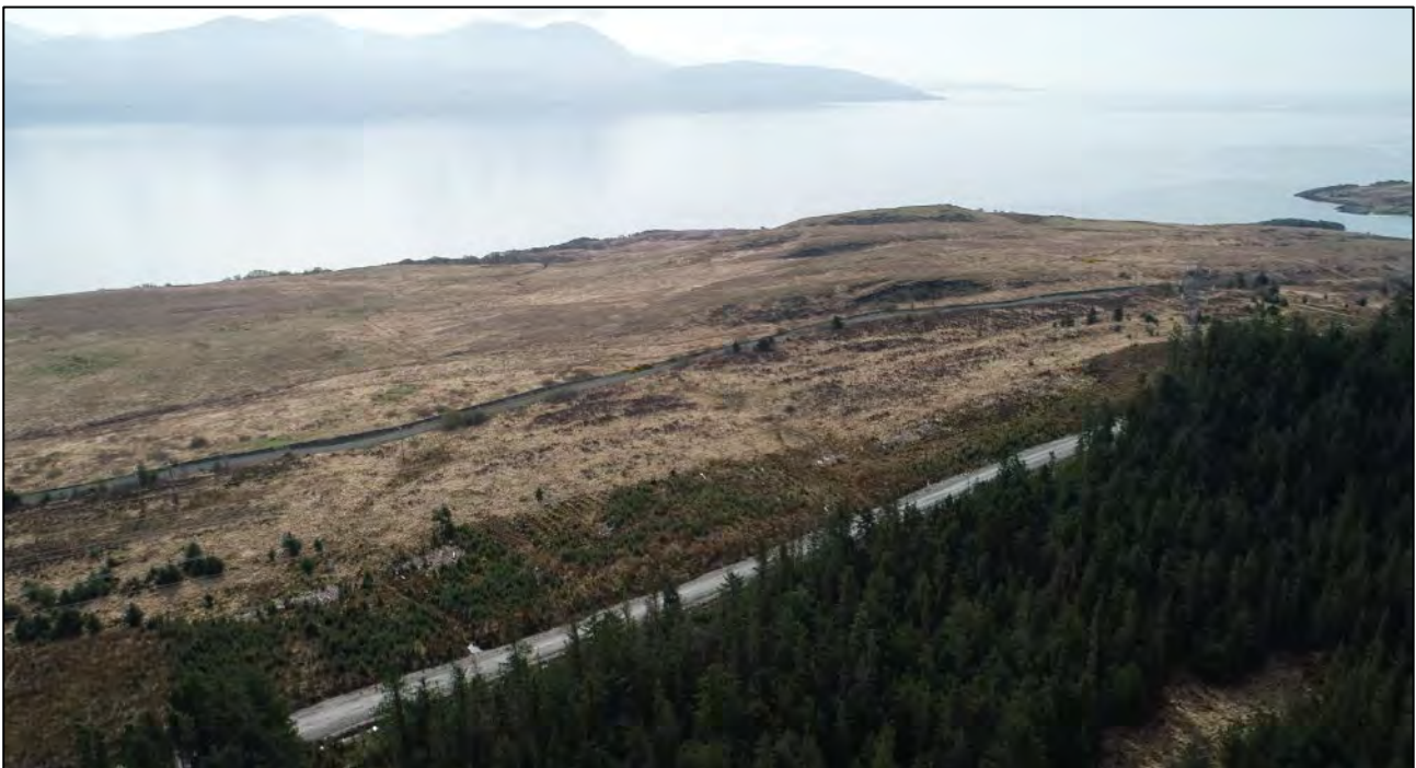
Plate 11 – View southeast showing part of the upgraded access track that falls within the red line boundary across the Crossaig and Cour estates towards the Kintyre haulage road (image taken from drone footage). The B842 is shown behind the access track.
