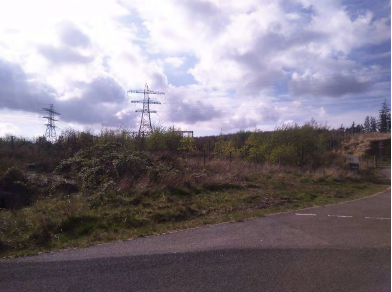
Plate 14 – Looking north-west towards the Proposed Development from the existing Crossaig substation bellmouth on the B842.
