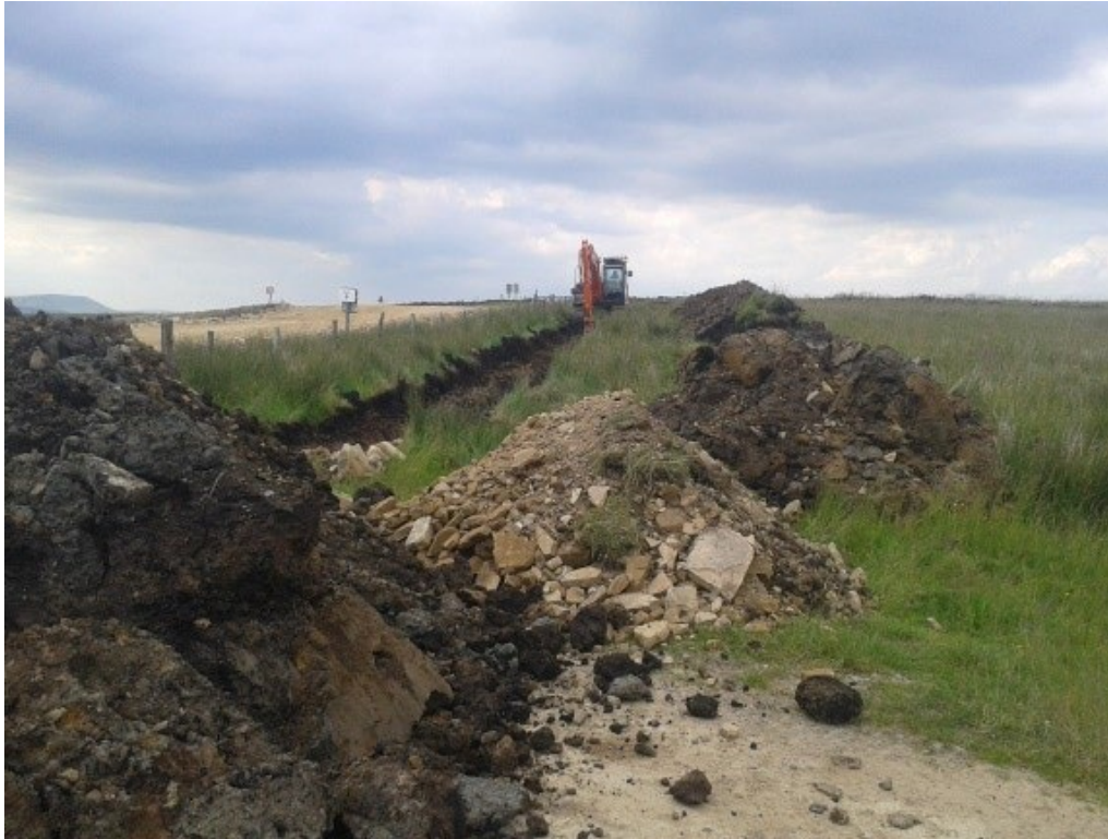
Plate 3.1: Stockpile and drainage ditch (under construction)
