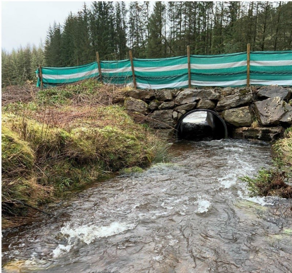
Plate 3.4: Silt Fencing at Watercourse Crossing
