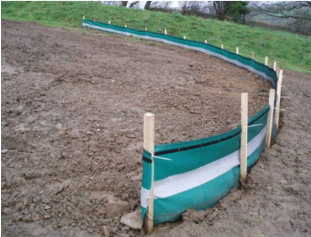
Plate 3.4: Silt Fencing at Watercourse Crossing
