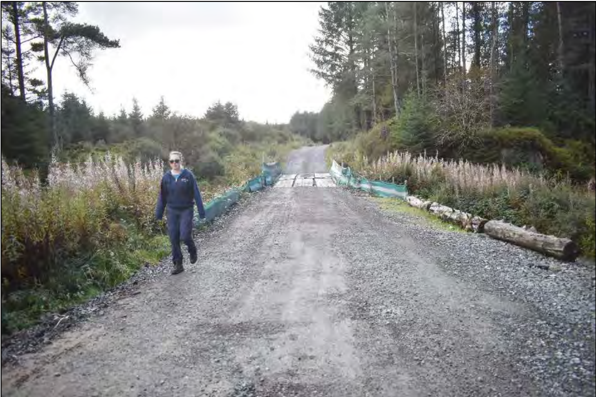
Plate 15: Location of bridge CR03, facing southwest
