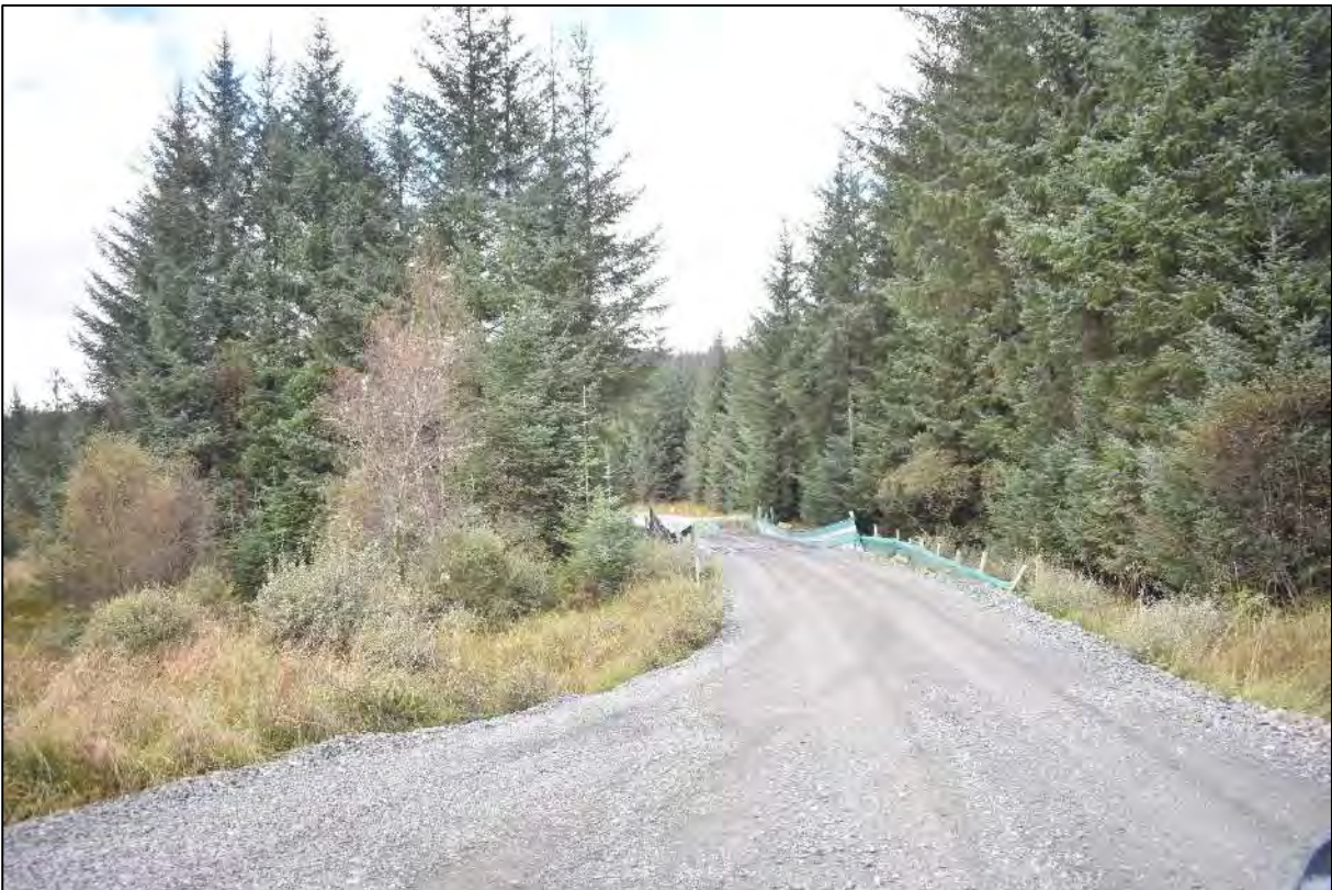
Plate 16: Location of bridge CR05, facing northwest
