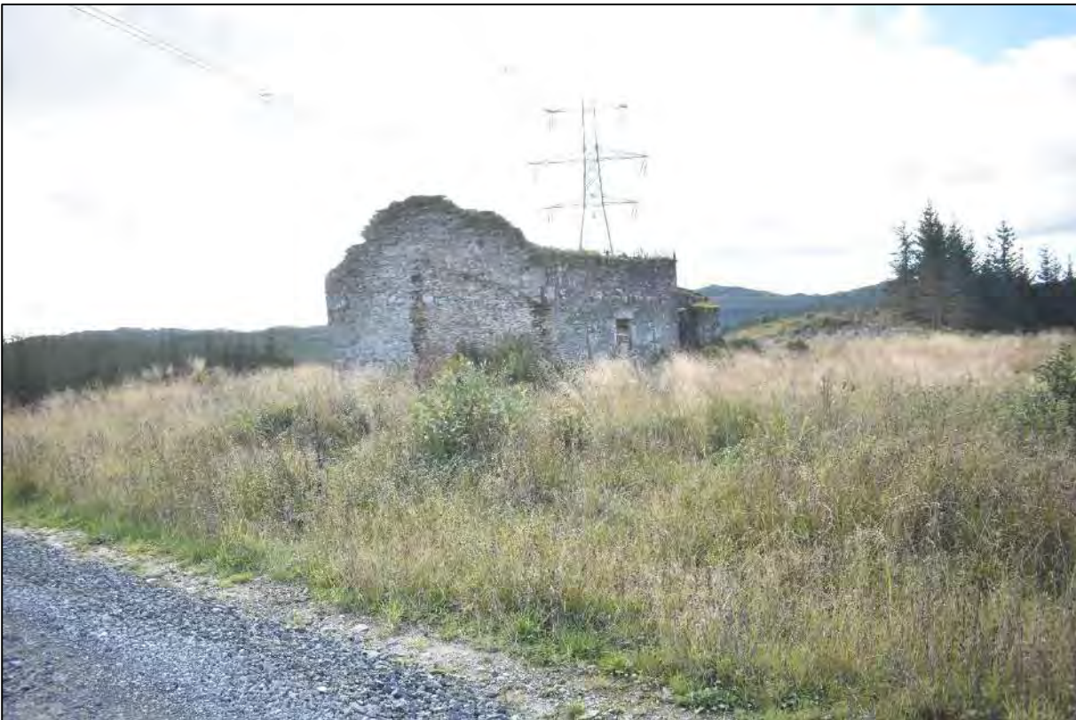
Plate 14: Location of settlement asset CR04, facing southwest
