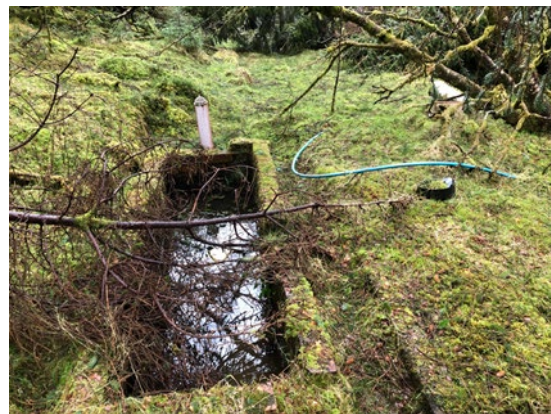
Plate 3.2 PWS source structures for PWS Crossaig Lodge and South Crossaig, NGR: NR 82848 50643 (Left: old weir intake pipe which is broken, right: debris covered weir tank with blue pipe disconnected from tank).
