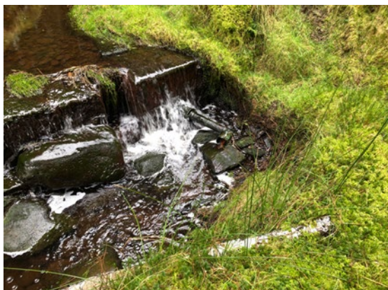
Plate 3.2 PWS source structures for PWS Crossaig Lodge and South Crossaig, NGR: NR 82848 50643 (Left: old weir intake pipe which is broken, right: debris covered weir tank with blue pipe disconnected from tank).
