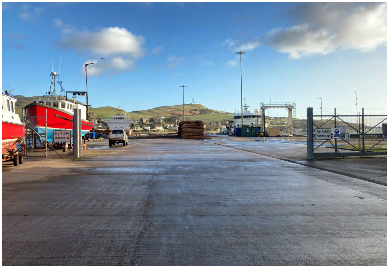
1a. Exit Campbeltown Harbour.
