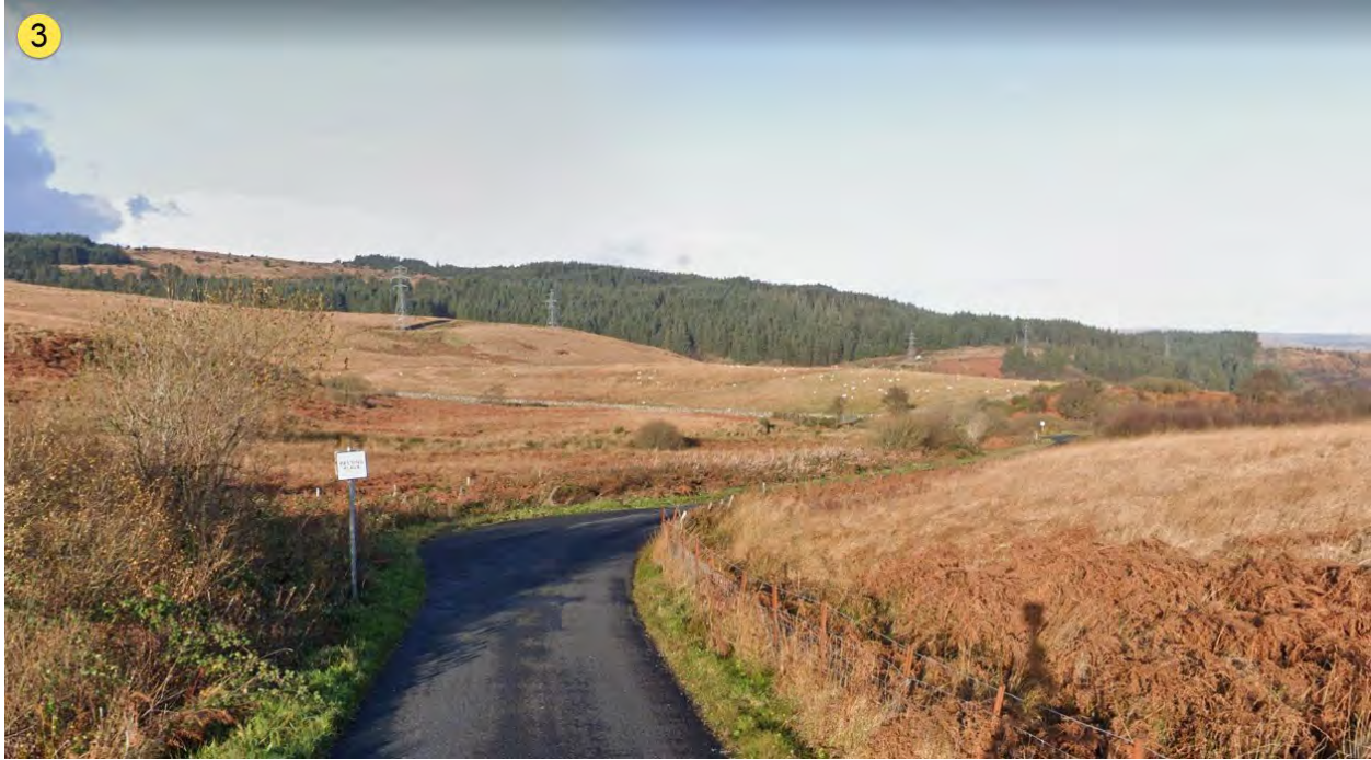
Road widened on nearside.
