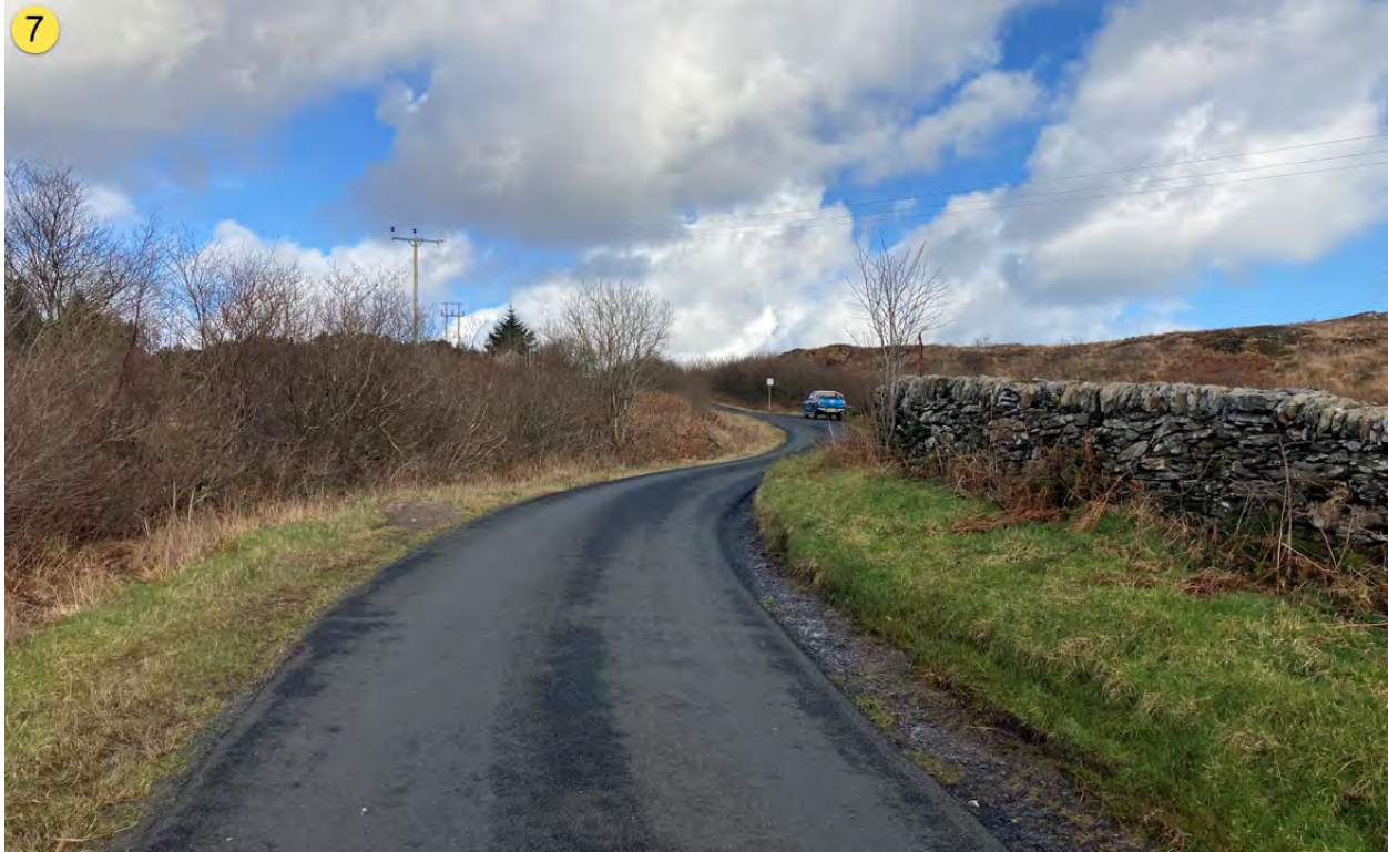
Road widened. Wall may need to be temporarily reduced in height.
