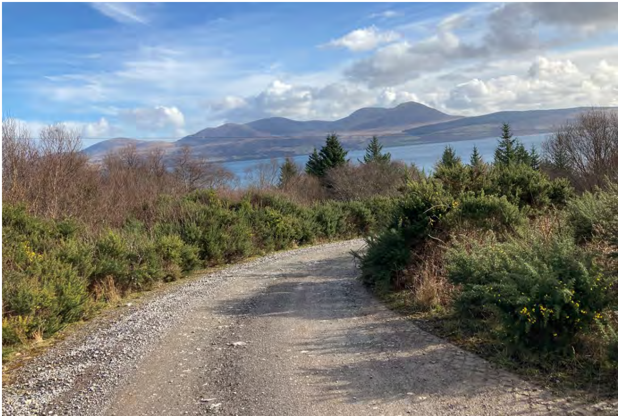
5b. Road will require widening on nearside and vegetation removed on offside.
