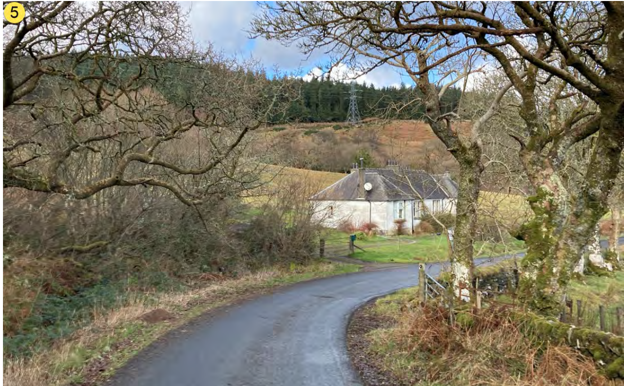
Road widened both sides. Vegetation/tree removal. And fence/post realigned.
