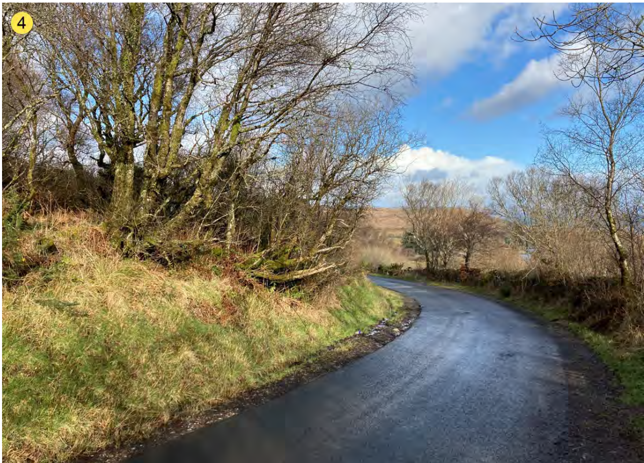
Road widened offside. Vegetation removed and bank regraded.
