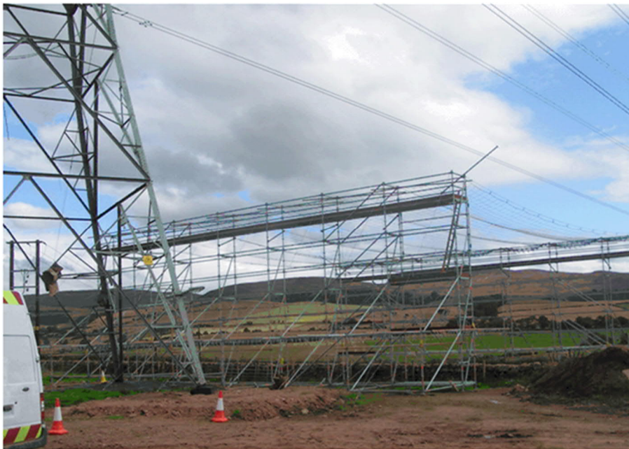
Photograph 2.3 Illustrative Image of Temporary Construction Scaffolds
