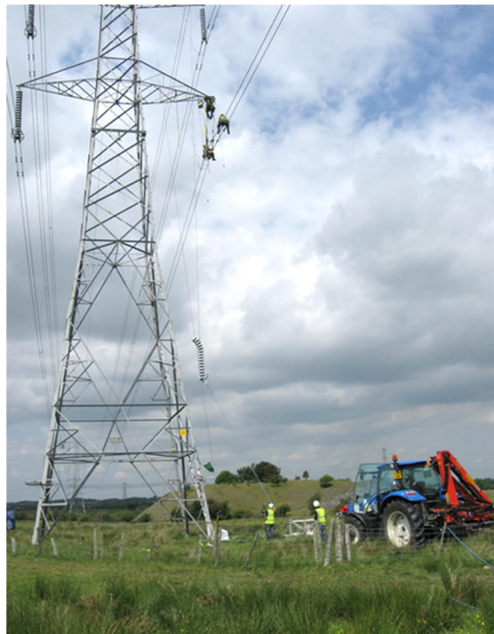
Photograph 2.2 Replacing insulators on an existing OHL tower
