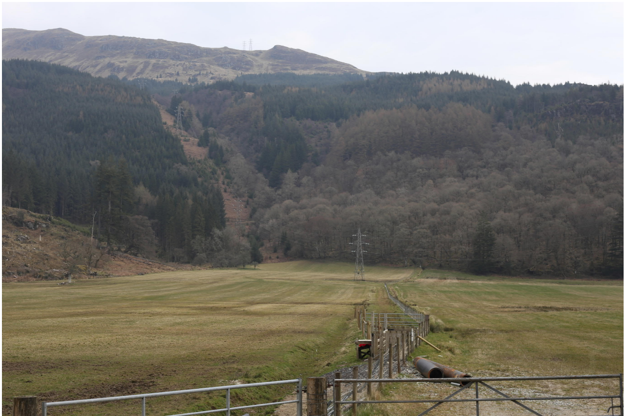
Plate 4.4: View from bridge over Glen Finart burn looking north-east towards the existing OHL and proposed Helicopter Operations Compounds.
