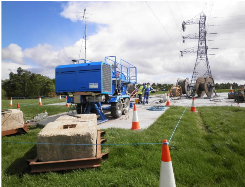
Photograph 2.1 Typical EPZ with equipment set up for re-conductoring
