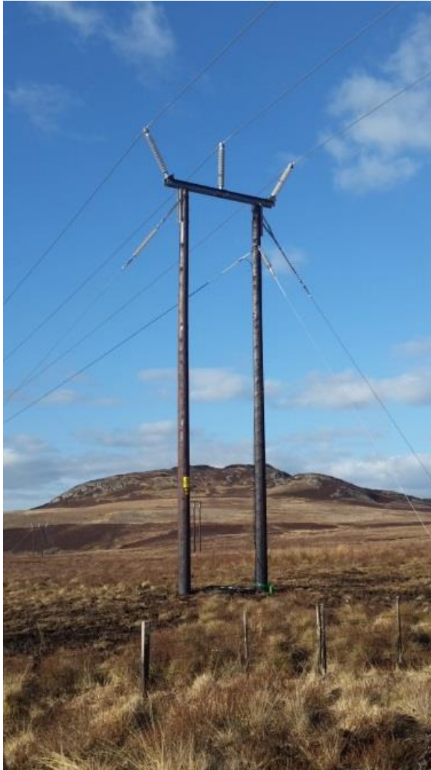
Plate 2.1: Wood Pole Trident Configuration
