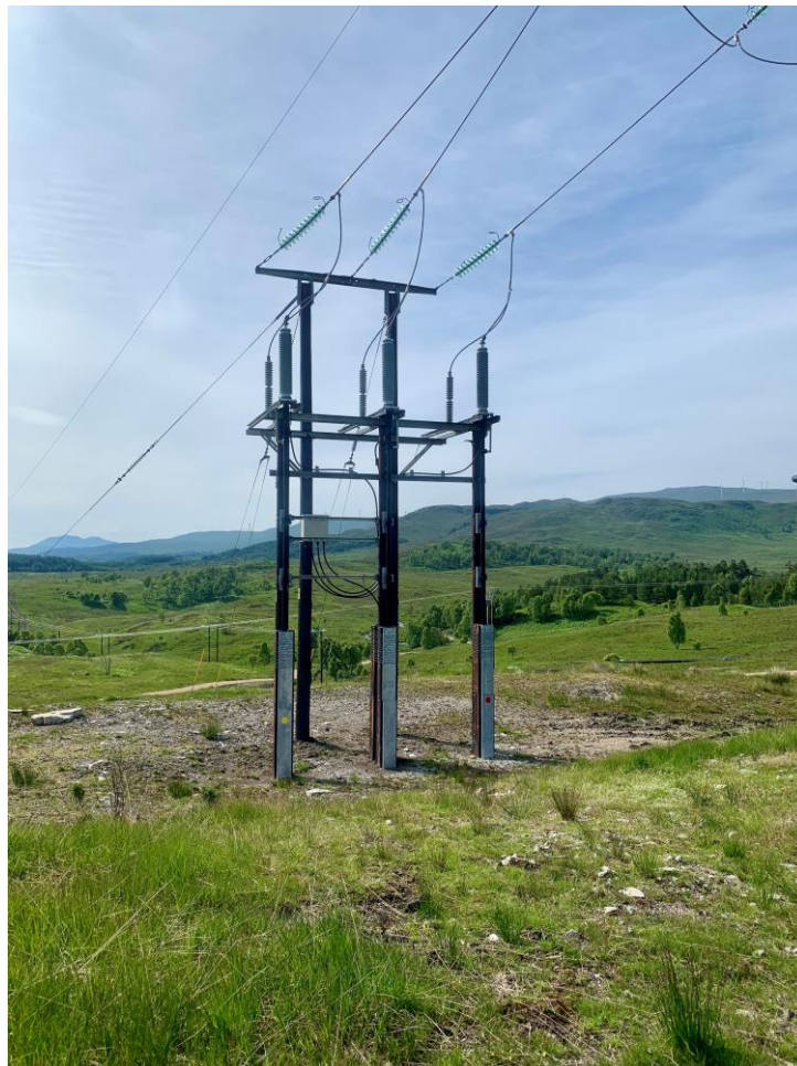
Plate 3.2: Typical Cable Sealing End Structure
