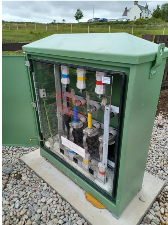
Plate 3.3: Typical Link Pillar
