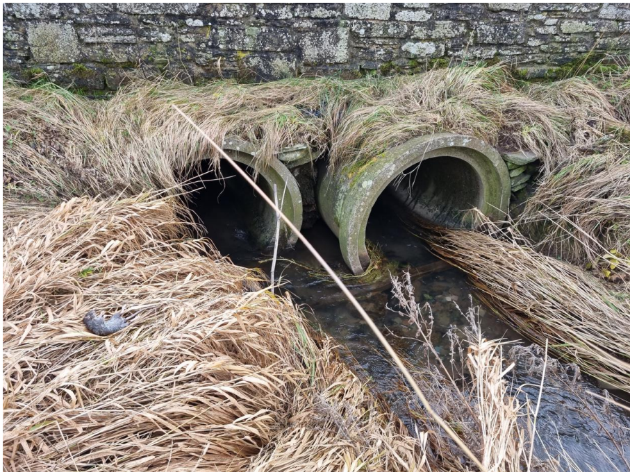
Photo 5.3: Twin culverts under Emmock Road
