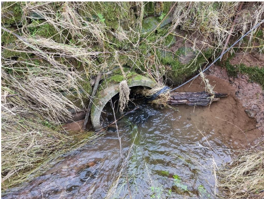
Photo 5.2: 0.450m culvert at T6-5
