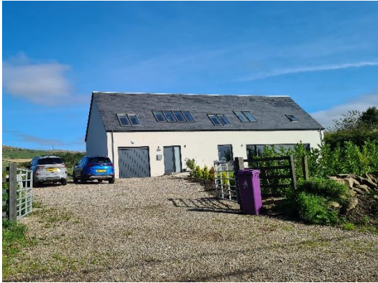
Principal elevation of Hillview House orientated to the south
