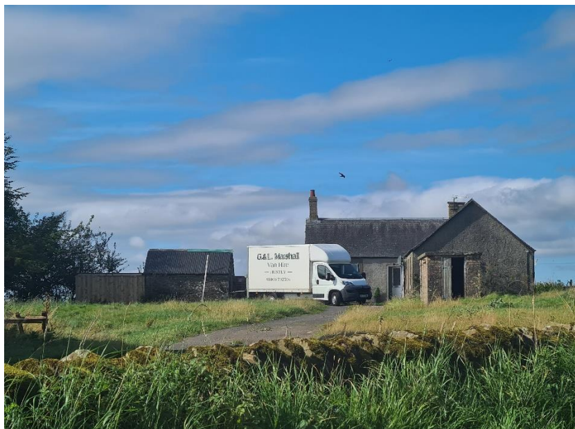
View looking west towards the eastern elevations of the property
