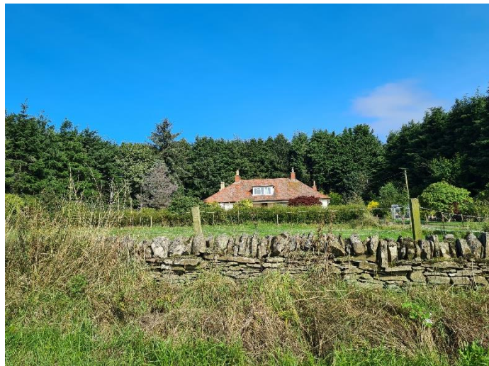
Principal elevation of property orientated to the south
