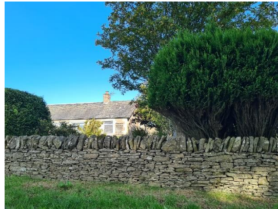
Principal elevation of 5 Balkemback Farm Cottages orientated to the south with evergreen hedgerows and stone wall along southern curtilage boundary
