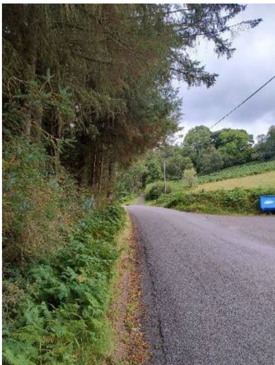
Figure 17: Public Road B852 looking north
