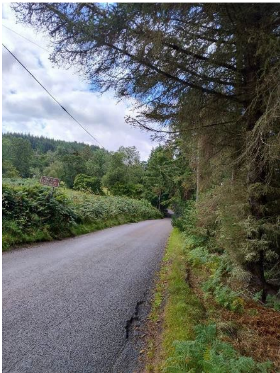
Plate 16: Public Road B852 looking south
