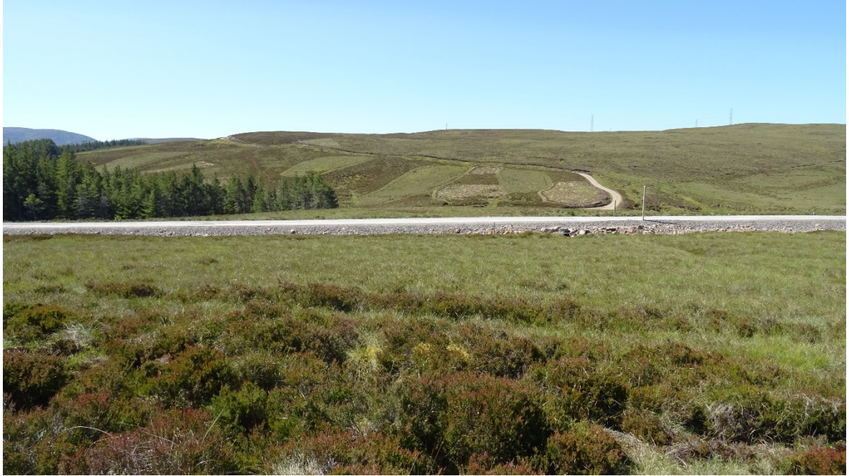
Photograph 2 - Floated Road near Proposed Glen Kyllachy Substation
