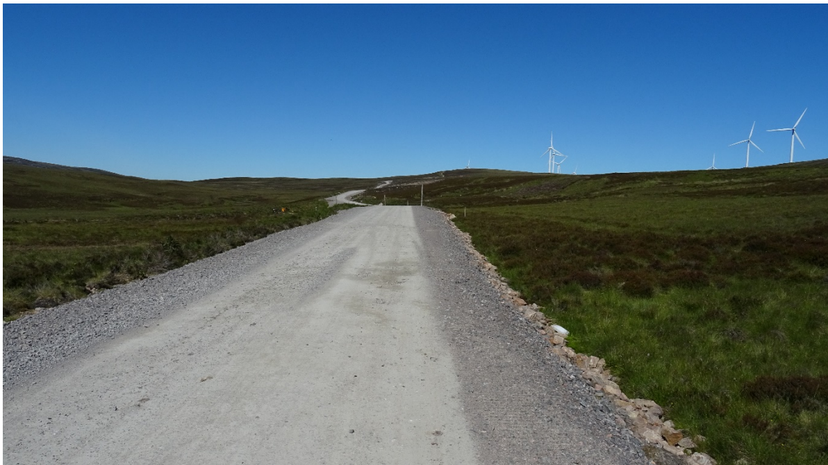
Photograph 1 – Looking towards proposed location of Glen Kyllachy Substation and Windfarm
