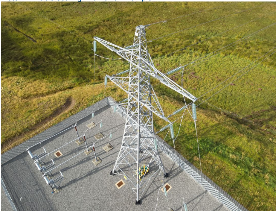
Plate 2.2: Cable Sealing End Tower Example
