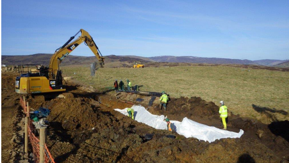
Plate 2.1: Example of Typical Cable Trench Excavation
